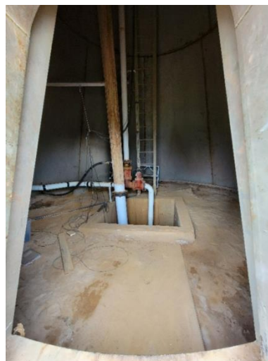
Interior tank near well #4
