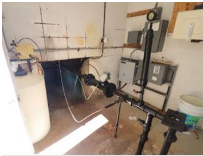
Interior of Well #2 well house.
