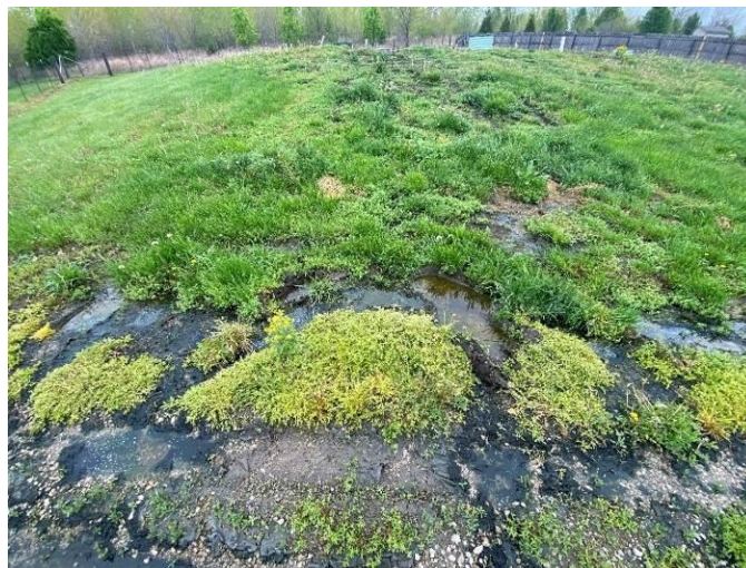
SSO at Berkshire Glenn (in background) due to sludge clogging filter bed
