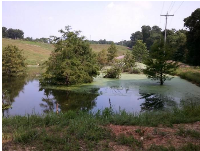
Trees growing and rotting in Port Perry lagoon cells
