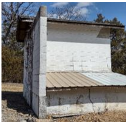
Well #2 site with vegetation removed
