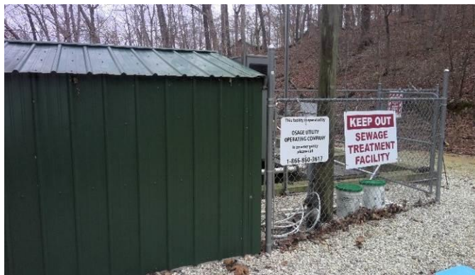
New blower housing and fence area
