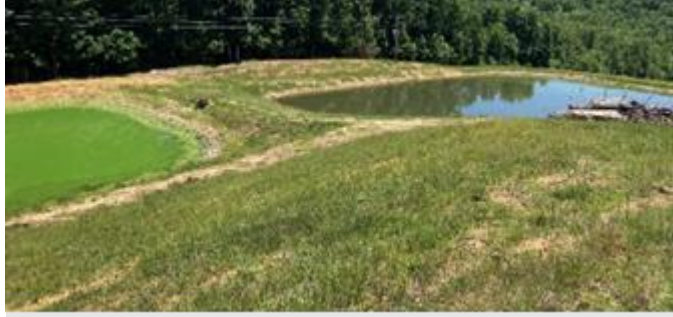
Lagoon cells cleared of trees after acquisition at Port Perry
