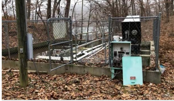
Overview of facility at acquisition
