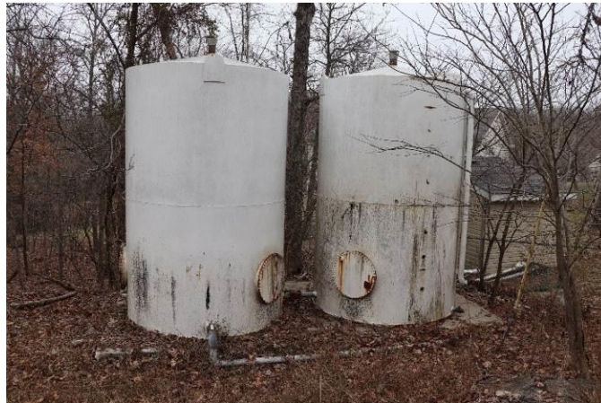
12 Condition of ground storage tanks at acquisition
