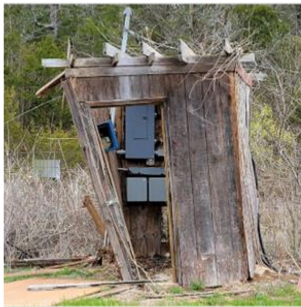
Condition of power/control structure at acquisition
