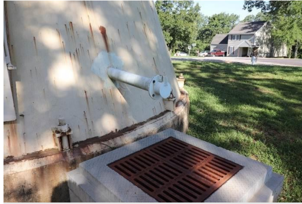
Base of tank near well #4
