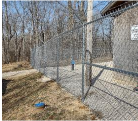
New fencing, gate, gravel and access road at Well #1
