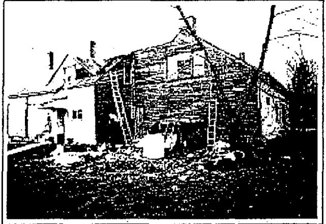
Movement of deteriorated foundation walls has opened large paths for air leakage.
