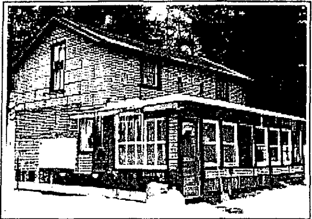
An uninsulated attic and air leakage between the porch and main structure are the main energy problems with this dwelling.
