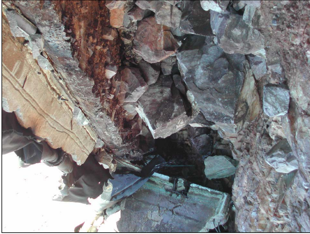
Rockfill between top of rock and base of plinth
