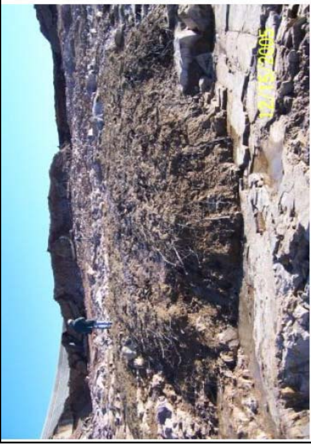
Eroded foundation, note rock jointing and overlying clay materials
