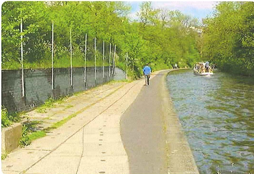
275 kV cables installed in surface troughs along tow path.
