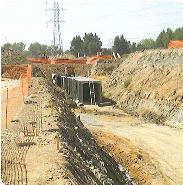
Cut and cover tunnel installation in mainland Europe. This technology is not used by National Grid.
