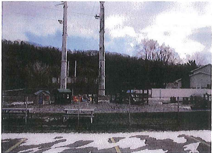
A preschool playground is located in a 161-kV transmission line easement in western Wisconsin. The house is approximately 25 feet from the edge of the easement.
