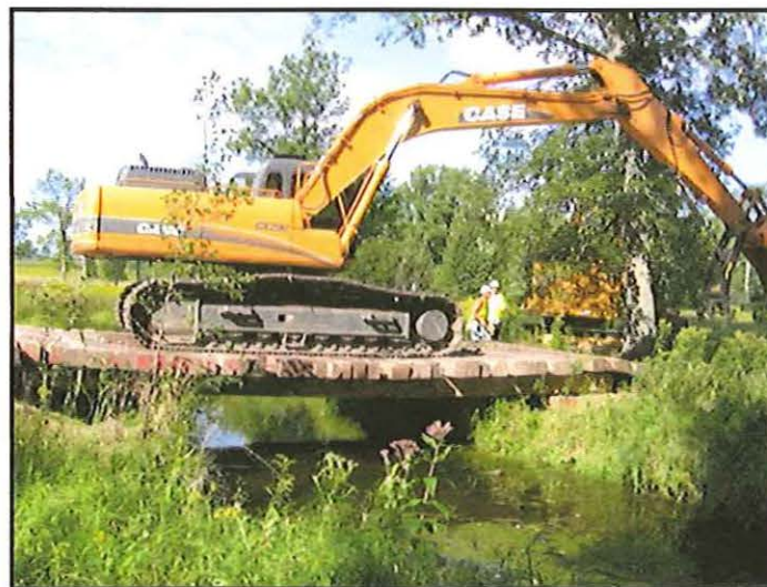
Figure 5 Temporary Bridge Structure Spanning a Waterway
