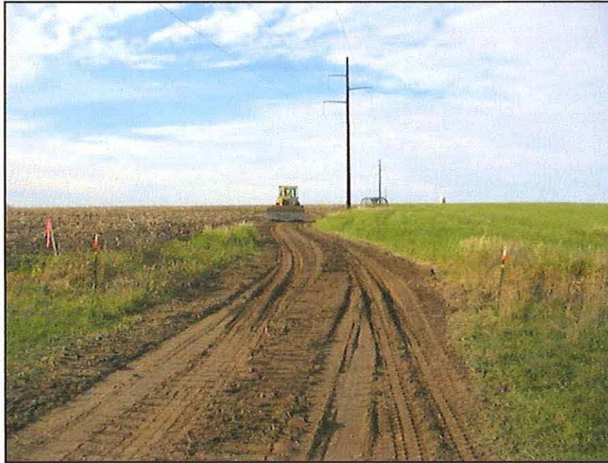
Figure 4 Smoothing Out Ruts by Backblading with a Dozer
