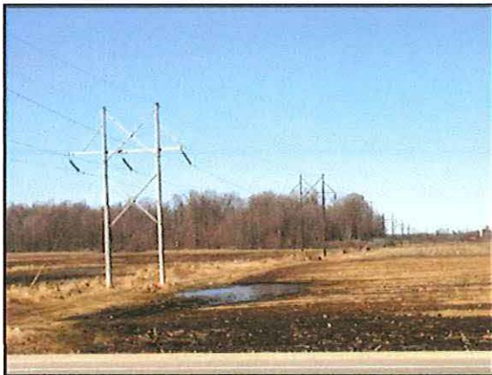
Figure 1 Typical Two-Pole, H-frame Structure
