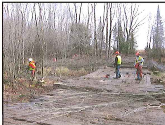
Figure 10 Hand Clearing Channel
