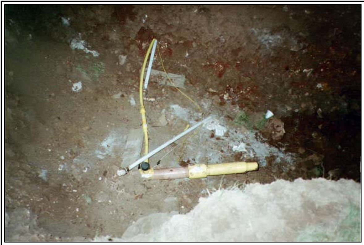
Photograph 4: View of the new natural gas PE piping that was installed on the evening of 9/25/02 to restore natural gas service to 1910 E. Burntwood Street.
