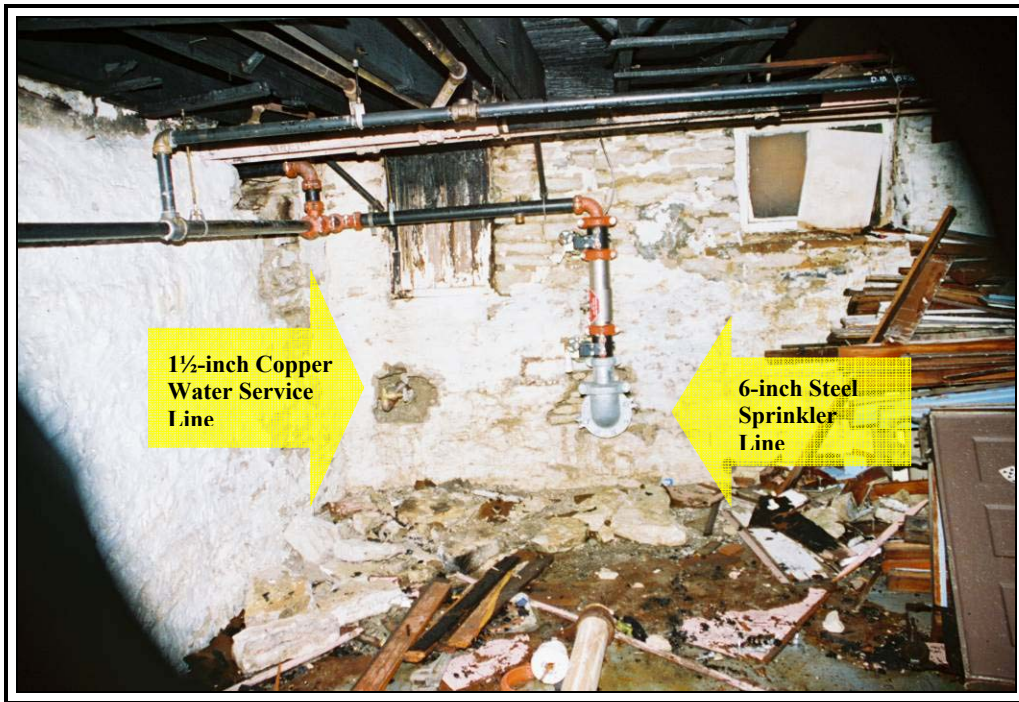
Photograph 5 View looking towards the south interior basement wall of 7527 Michigan Avenue where the 1½-inch copper water service line (to the left) and 6-inch steel sprinkler line entered. Note the burn damage to the wooden floor joists and the first floor flooring above.
