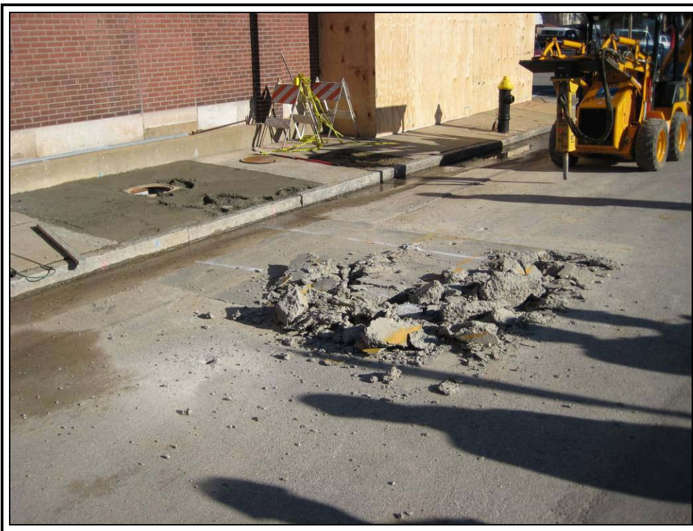
Photograph 2 View looking approximately to the east at the south wall of 7527 Michigan Avenue. The pavement in the street along Steins Street was broken in this location to access the Company's 4-inch natural gas CI main. Observe the freshly poured concrete sidewalk in the foreground along the south wall of 7527 Michigan Avenue.
