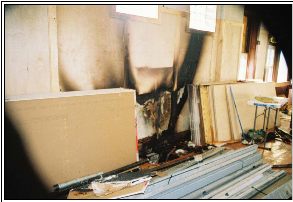
Photograph 6 View looking approximately to the southwest at the south wall of the first floor room inside of 7527 Michigan Avenue. A portion of the floor (located between the two stacks of sheet rock that were placed against the wall) was removed during fire suppression activities and a portion appeared to have been consumed by the fire. Observe the v-pattern burn that appears along the wall and above the opening in the floor.
