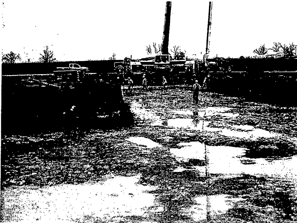
First Lean Concrete Mud Mat Poured: 1/04/2005
