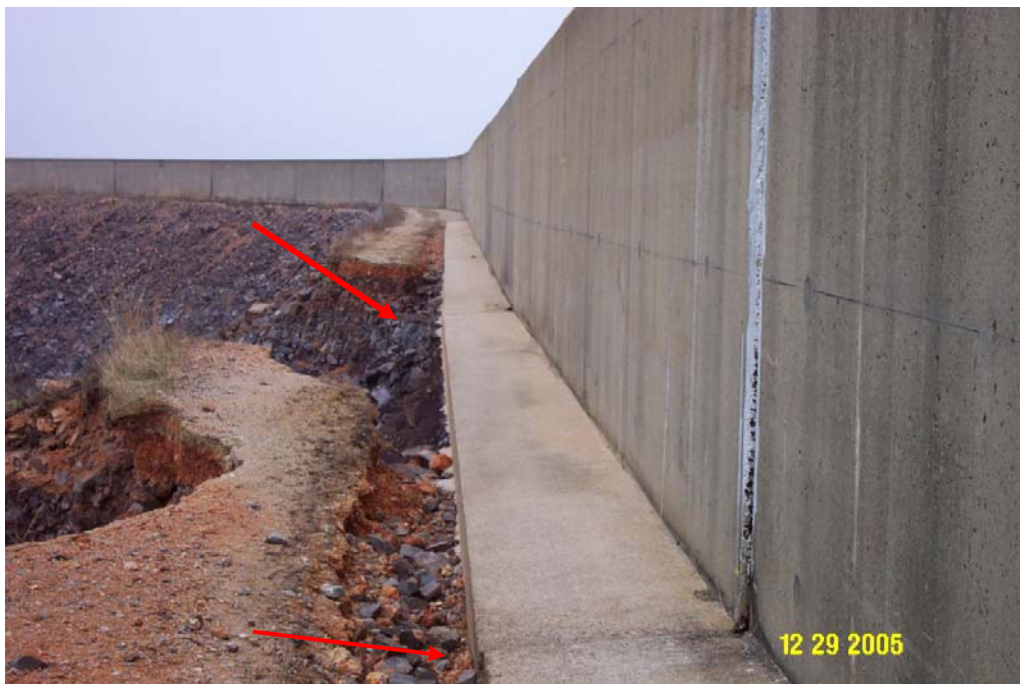
Figure 4.8 - Erosion at Panel 71 footing Note the horizontal displacement between Panel 70 and 71(foreground) and bowing at the joint between Panels 71 and 72. Erosion at the footing is similar to that described during the September 25, 2005 wave overtopping.
