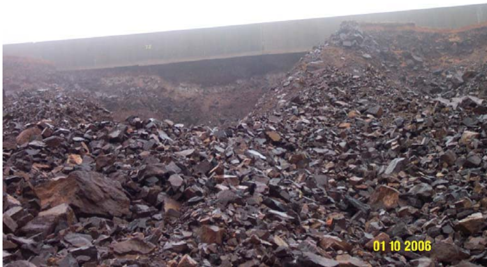
Figure 4.7 - Panel 72 Note erosion deep beneath the parapet wall Damage judged as significant Estimate 0.7 ft of overtopping
