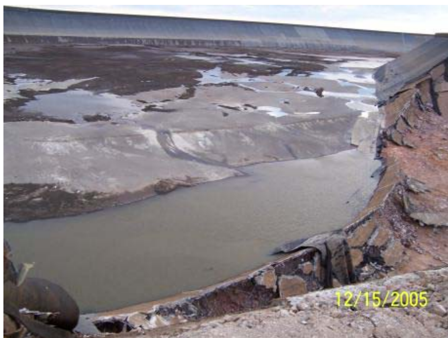
Figure 2.10 - Breached area. Note “fish pond” area immediately upstream of the breach. This area was over-excavated during original construction due to poor foundation conditions.
