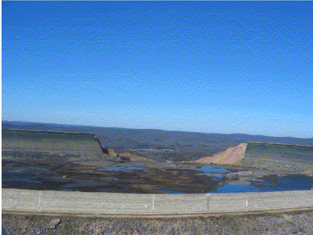
Figure 4.10 – Breach Panels 88 - 99 removed during the event Estimate 0.2 -0.3 ft. of overtopping. (Missouri DNR Photo)
