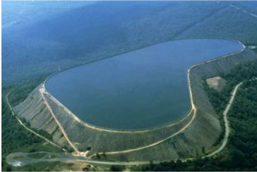
Figure 2.3 - View of upper Reservoir.
