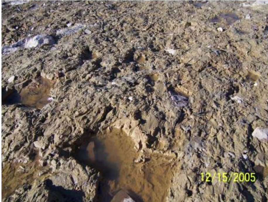
Figure 2.7 - Grooves cut into an area of clay-seam foundation by the floodwaters. This area is located immediately downstream and in the center of the breach.
