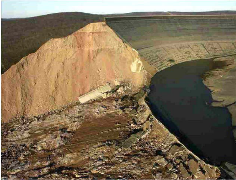
Figure 2.11 - Weathered rock and discontinuous clay seam foundation just downstream of fish-pond area.
