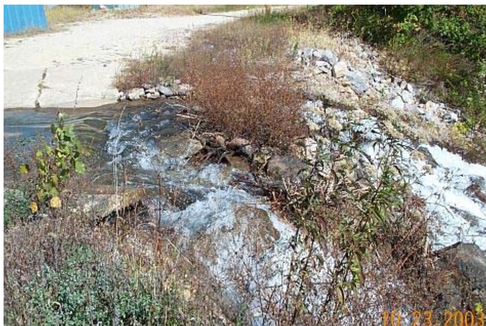
Figure 3.8 - Overflow of the seepage collection Pond before liner installation (2003 FERC Operation Inspection Report)
