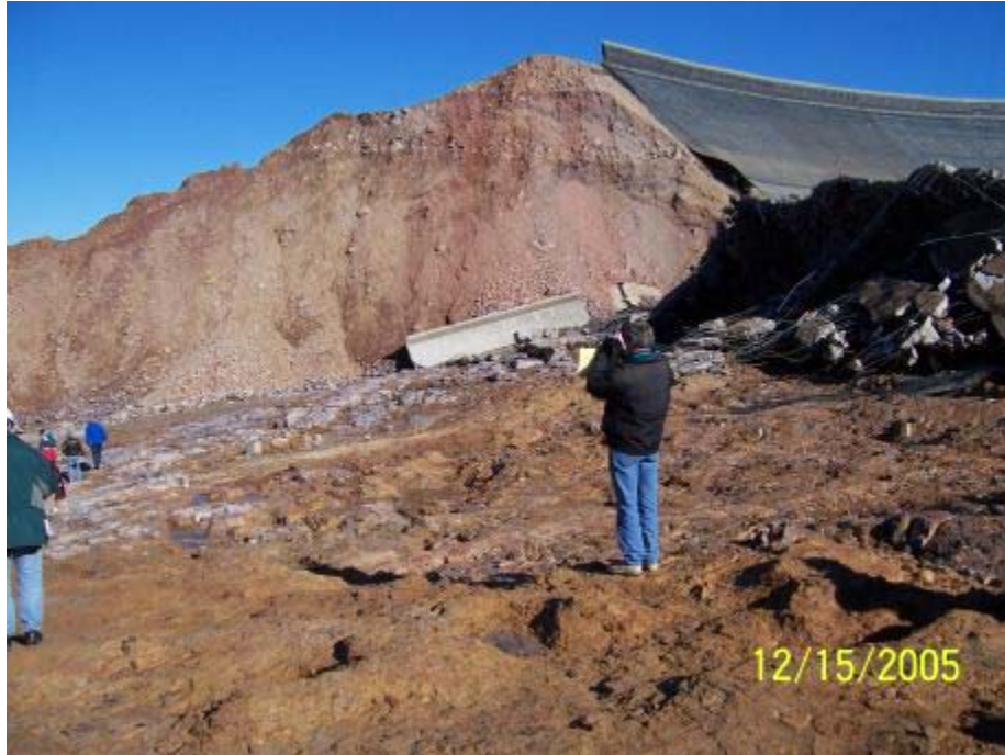
Figure 9.2 - Area of weathered rhyolite, which is in-line with the “fish pond” depression in the reservoir (background).
