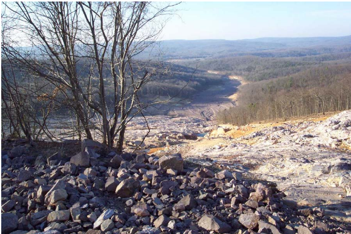
Figure 11.3– Downstream view from breach (Source: Staff, 12/22/05)
