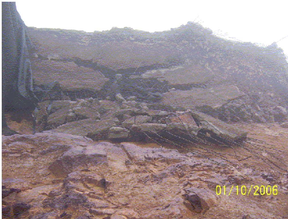
Figure 2.4 - View of bedrock immediately below failed embankment section. Note weathered clay in lower portions of the exposure.
