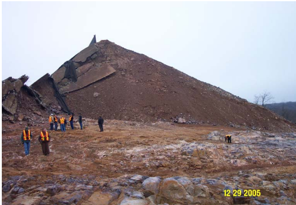
Figure 4.11 - Left side of breach
