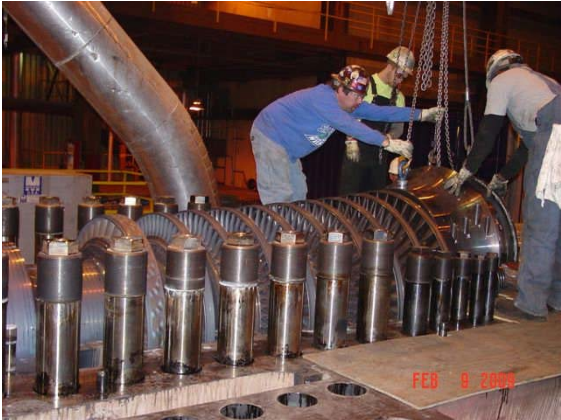
Removing UH N1 Packing Casing
