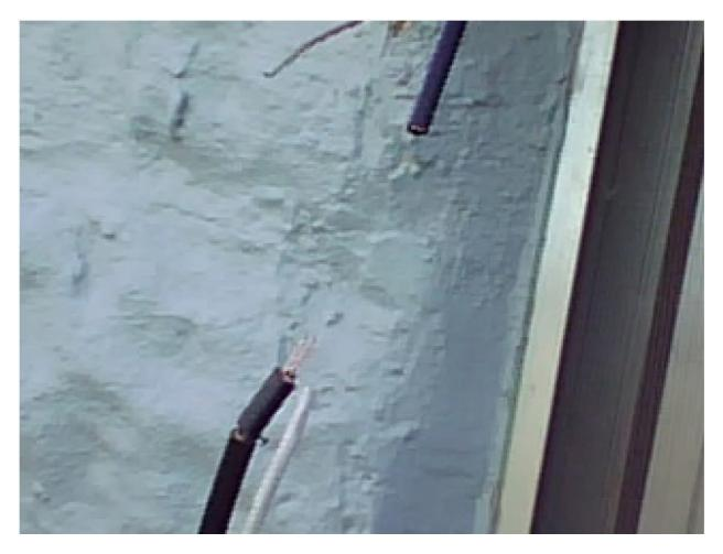
Photograph taken on October 9. 2008. Photograph shows CenturyTel drop wire and ground wire cut by Charter before attachment to the NID.
