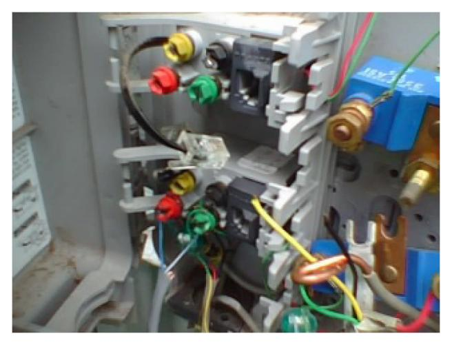
Photograph taken on October 7, 2008. Photograph shows CenturyTel ground wire and other internal NID connections ripped or pulled out. Charter connection (using the blue-green plastic connector) is just visible at the bottom of the picture.
