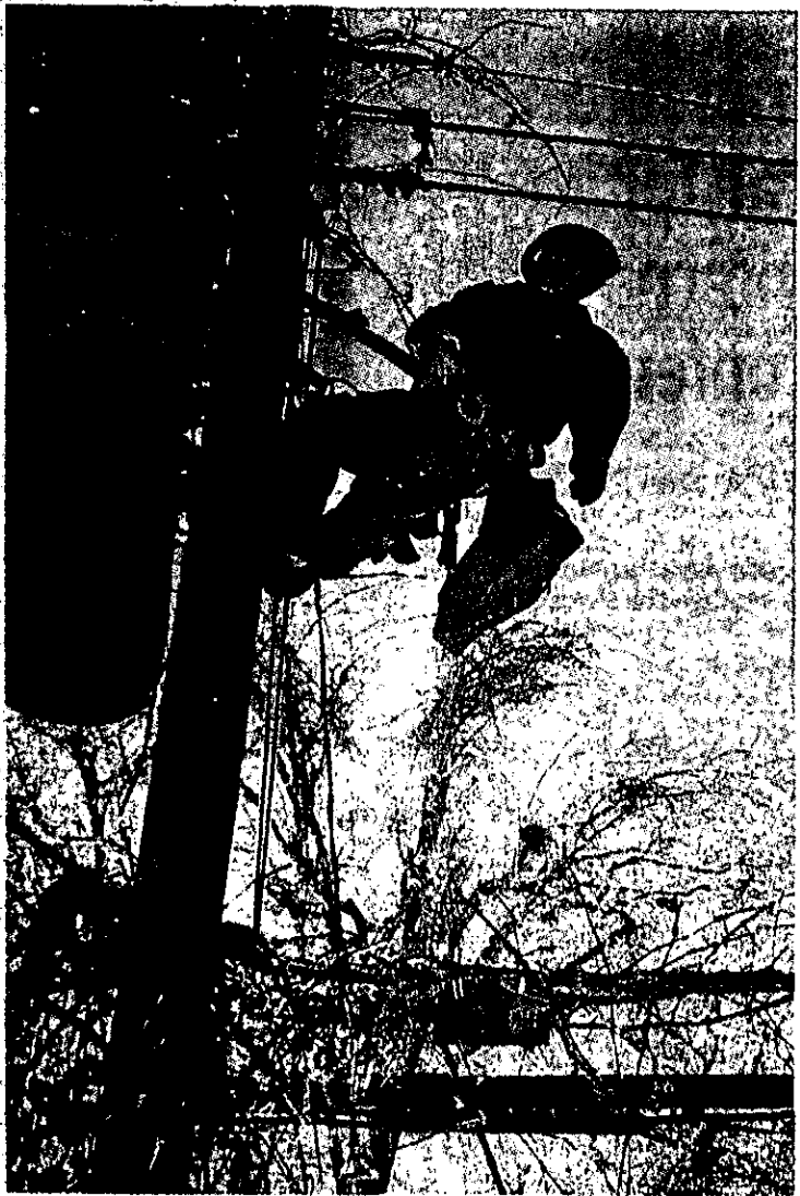
Kyle Giesler, an Ameren employee, waits for another worker to help repair the main power line behind a home at 78 Greendale Drive in Greendale, south of UMSL. In the background are trees still loaded with ice. Sam Leone | Post-Dispatch
