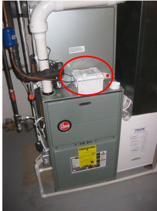
Figure 7. Cellular Logger (Completed Installation)
