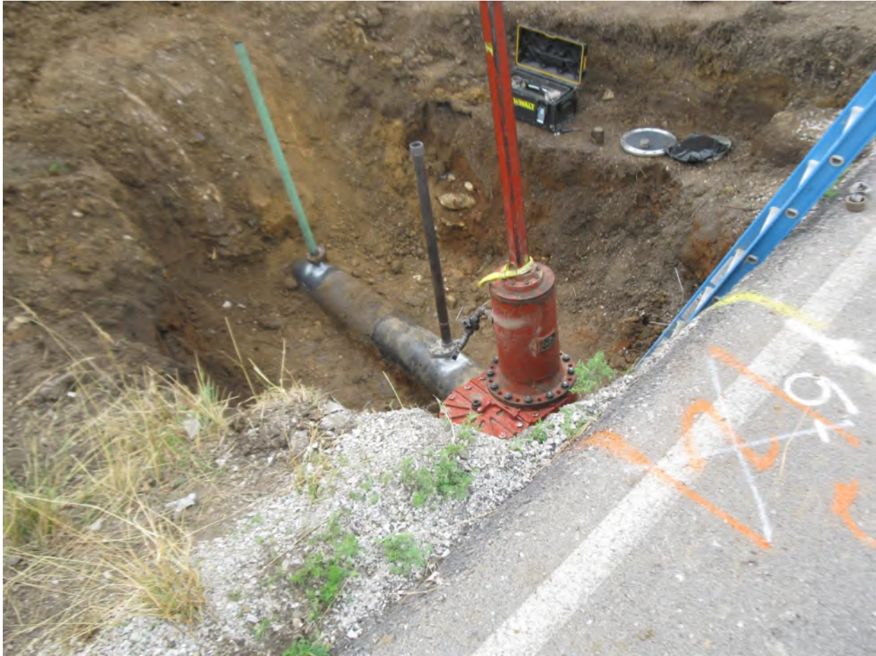
Photograph 2: Photograph of tapping and line stop fitting affixed to the pipeline on the west side of U.S. Route 169. (Source: Staff)
