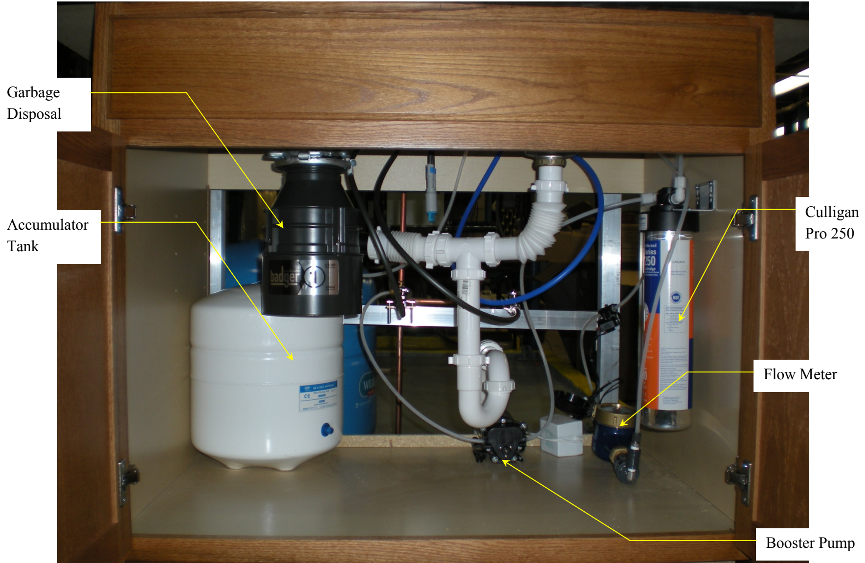
Figure 4-1. Typical Adsorption POU Undersink Installation
