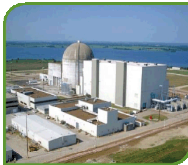
Wolf Creek Nuclear Plant – Burlington, Kansas
