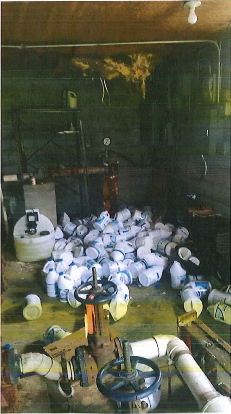
View of Hole Over Well Head (exposed wiring and insulation)
