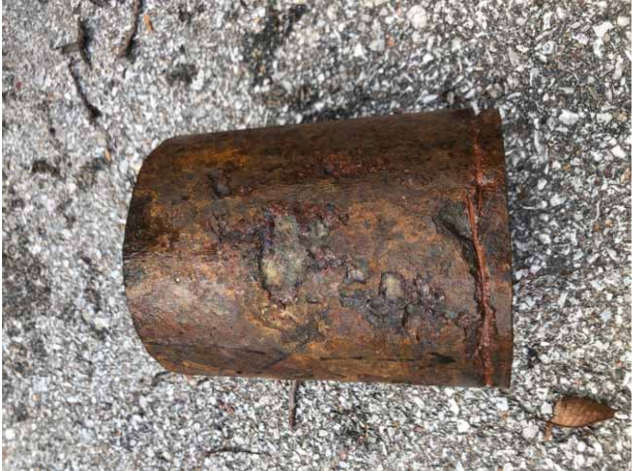
Figure 26, Spire East, South Region, Cast Iron, Work Order #171733652
