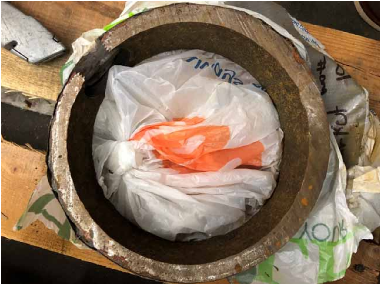
Figure 5, Spire East, North Region, Cast Iron, Work Order #19444783
