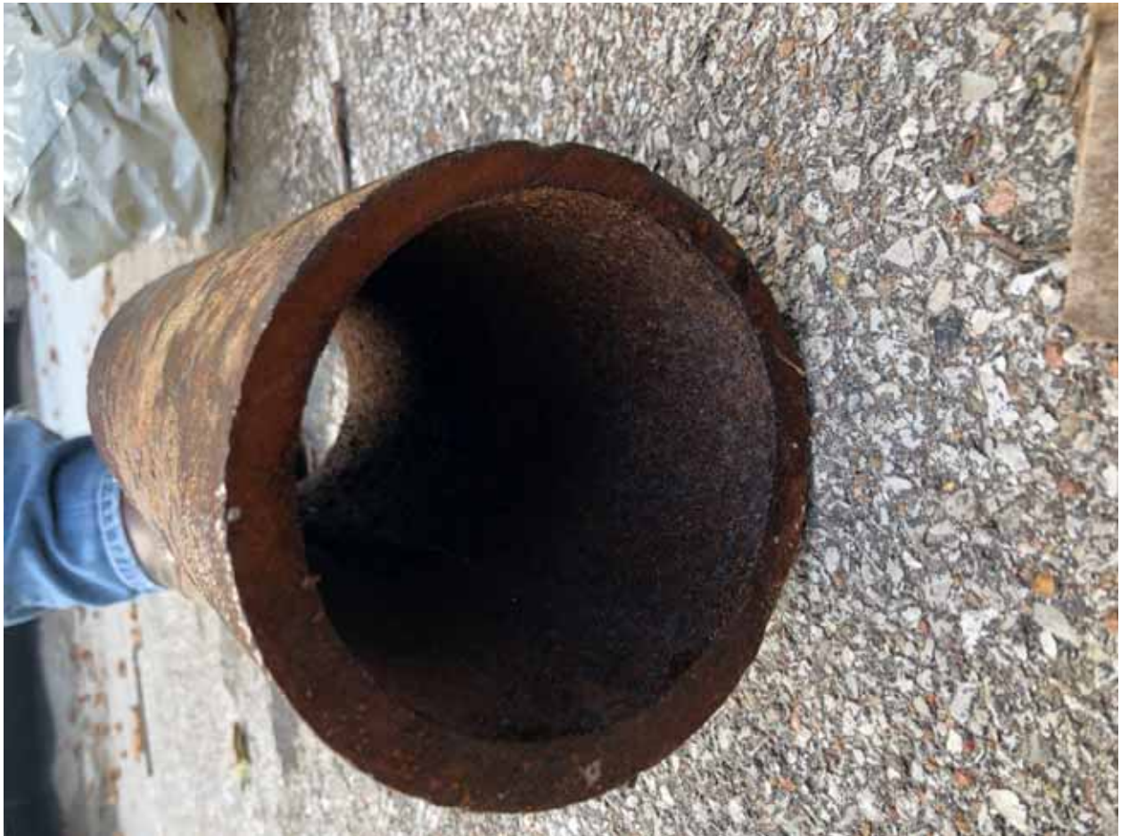
Figure 30, Spire East, South Region, Cast Iron, Work Order #171733652
