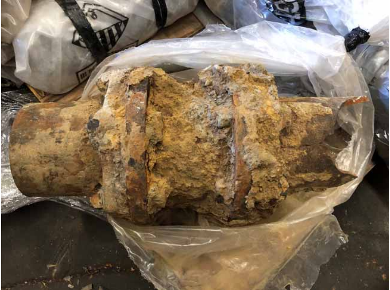
Figure 11, Spire East, North Region, Cast Iron, Work Order #20765542
