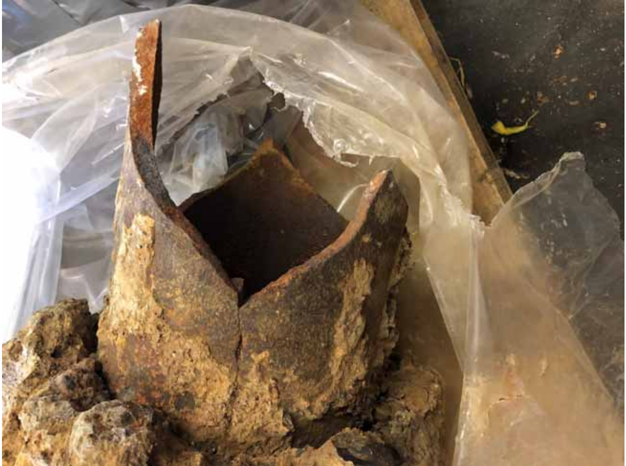
Figure 12, Spire East, North Region, Cast Iron, Work Order #20765542
