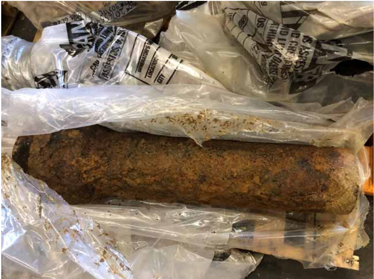
Figure 15, Spire East, North Region, Cast Iron, Work Order #20351410
