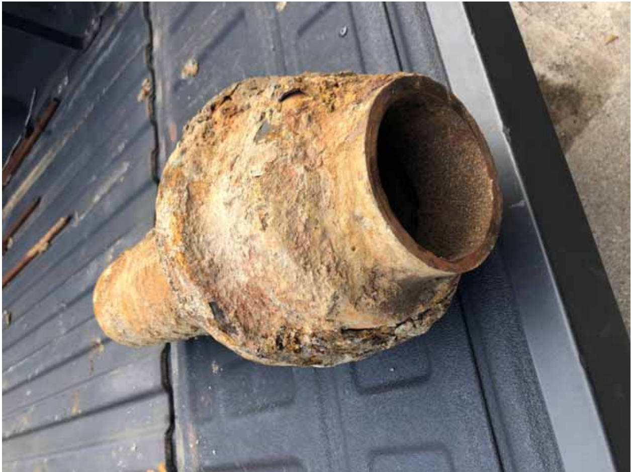
Figure 42, Spire East, South Region, Cast Iron, Work Order #196553364
