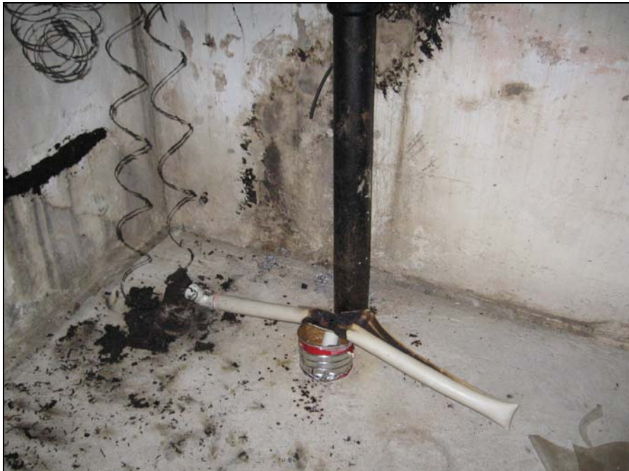
Photograph 2 Improperly installed sewer drain pipe and fire damage in the basement of 1706 SW Smith Street
