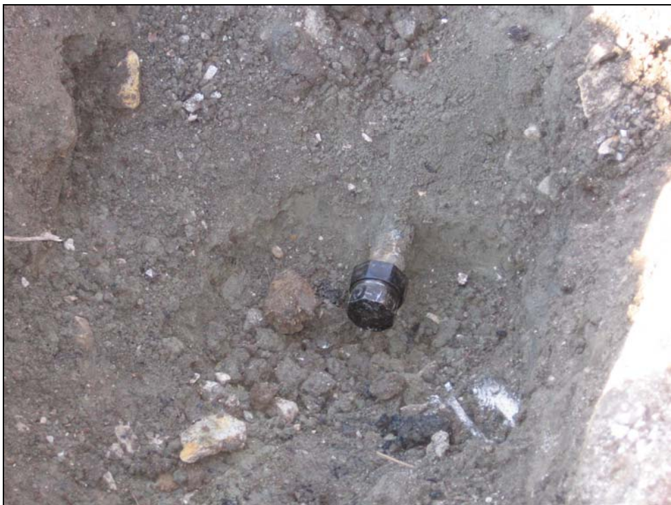
Photograph 2 Capped 2-inch abandoned natural gas main
