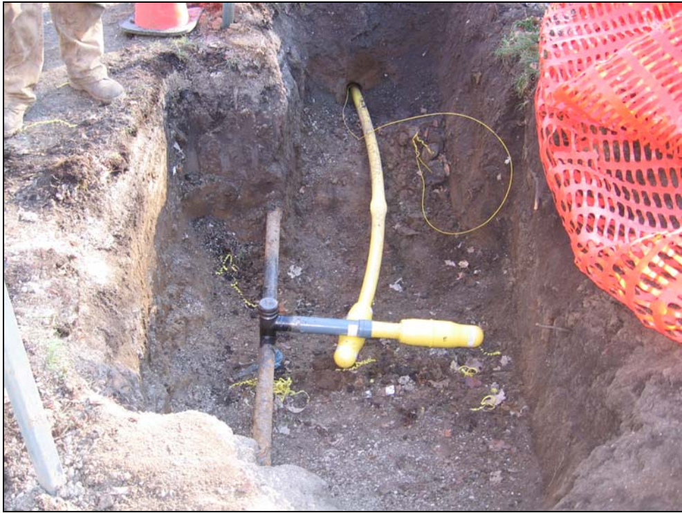
Photograph 1 Incorrectly tapped 2-inch abandoned natural gas main
