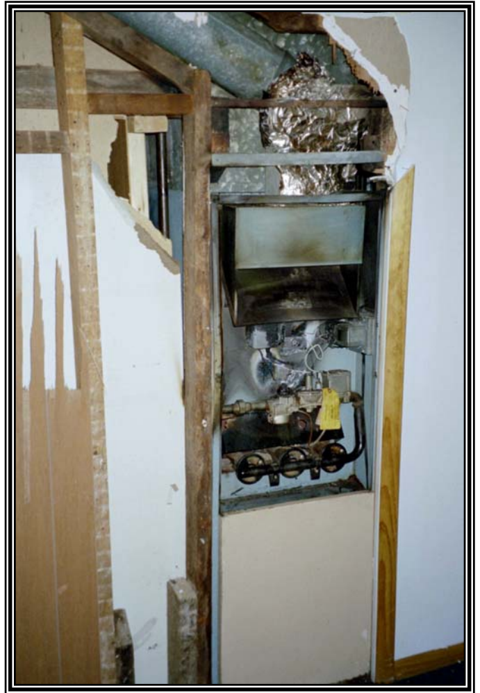
Photograph 5 Looking at the natural gas furnace for 1303 Nelson Street.
