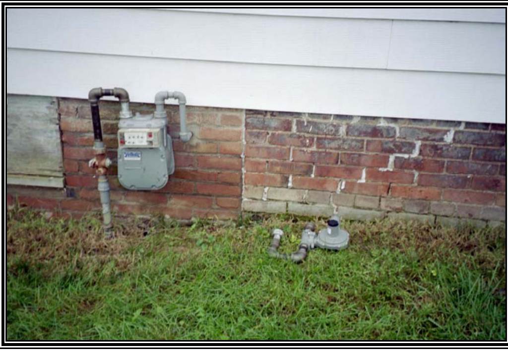
Photograph 7 Looking south at the natural gas meter that is located on the north side of 1222 6 th Street. Observe that no pressure regulator is installed due to the fact that the meter is connected to the low-pressure system. Notice the new service regulator that is lying on the ground.
