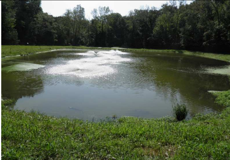
Photograph #: 1 Taken by: Stephen Moss Entity: BCSD, Trails West Subdivision Permit: #MO-0092002 Location: BOONE Description: View of the primary cell. The facility's aerators can all be observed in the picture and appear to be functioning properly. Date Taken: September 1, 2016 Program: WPC Unit
