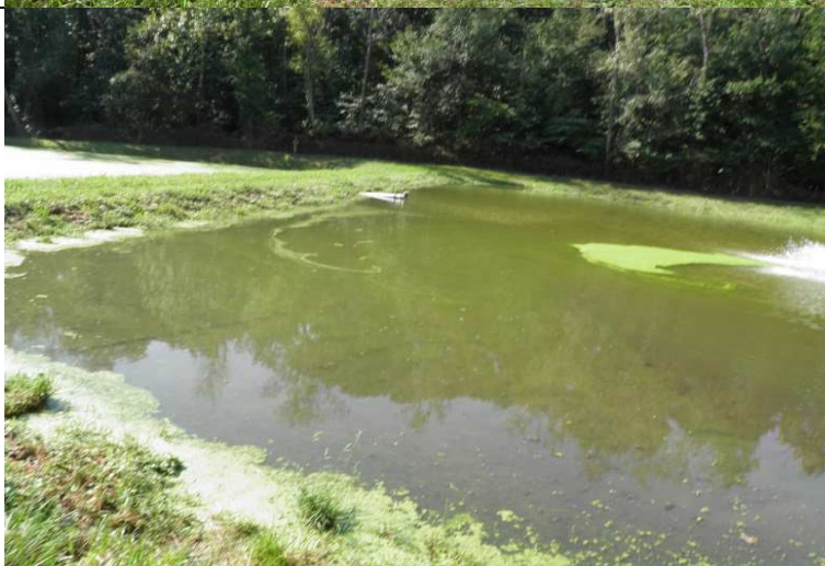
Photograph #: 3 Taken by: Stephen Moss Entity: BCSD, Trails West Subdivision Permit: #MO-0092002 Location: BOONE Description: View of the south side of the primary cell. The transfer pipe between the primary and secondary cell can be observed in the picture. Date Taken: September 1, 2016 Program: WPC Unit
