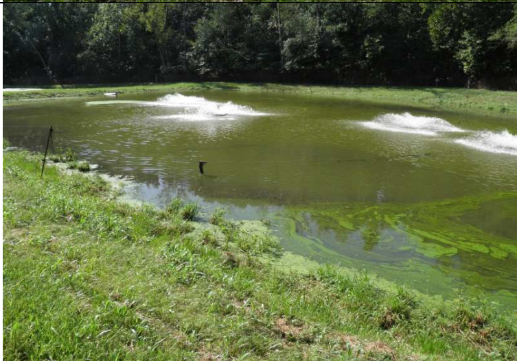
Photograph #: 2 Taken by: Stephen Moss Entity: BCSD, Trails West Subdivision Permit: #MO-0092002 Location: BOONE Description: View of the primary cell. Erosion damage can be observed on the inner berm slope of the lagoon. The aerators can also be observed in the picture and they appear to be functioning properly. Date Taken: September 1, 2016 Program: WPC Unit
