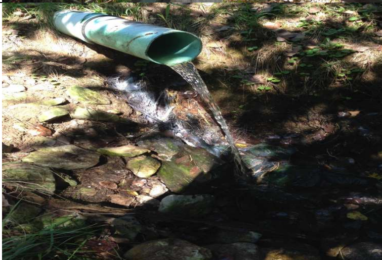
Photograph #: 6 Taken by: Stephen Moss Entity: BCSD, Trails West Subdivision Permit: #MO-0092002 Location: BOONE Description: View of Outfall #001. Hydrogen sulfide bacteria can be observed below the outfall pipe. Date Taken: September 1, 2016 Program: WPC Unit
