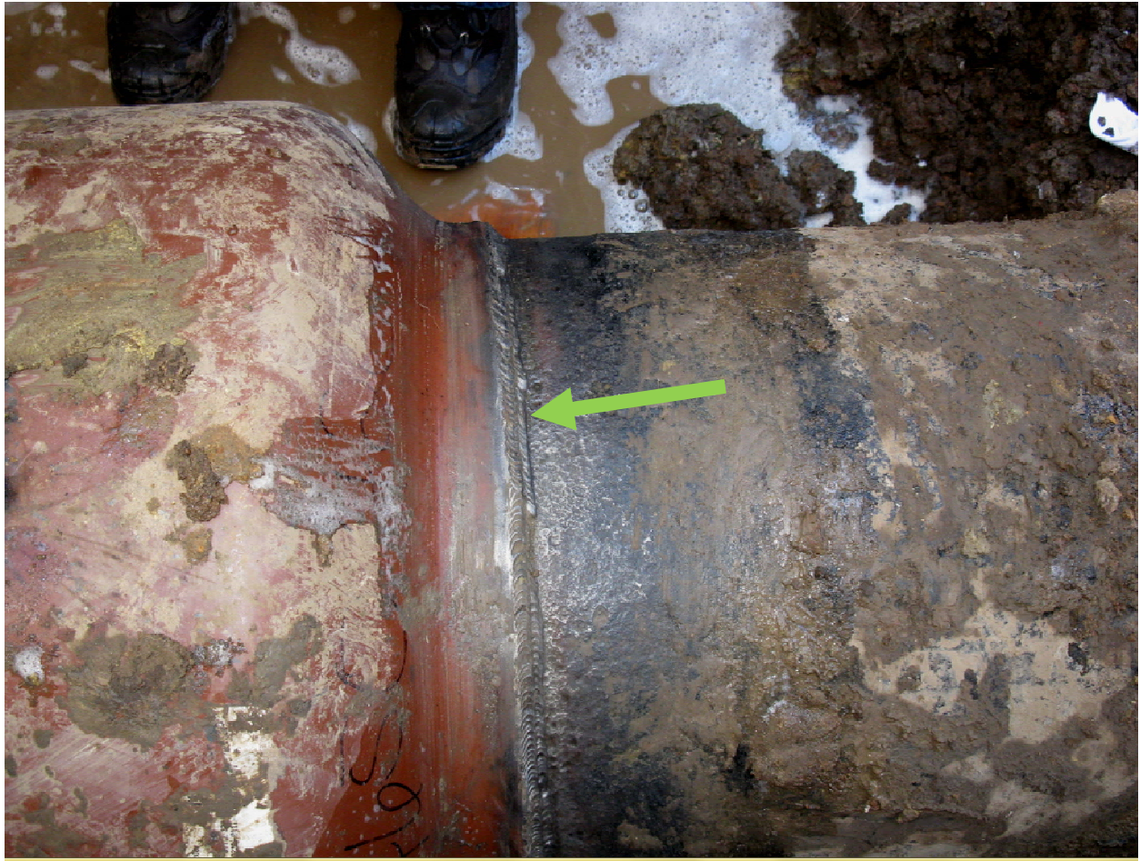
PHOTOGRAPH 3: Weld Bead (Arrow) joining Welded Repair Sleeve to Mayfair 16-inch pipeline (Staff Photo)
