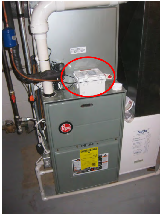
Figure 7. Cellular Logger (Completed Installation)
