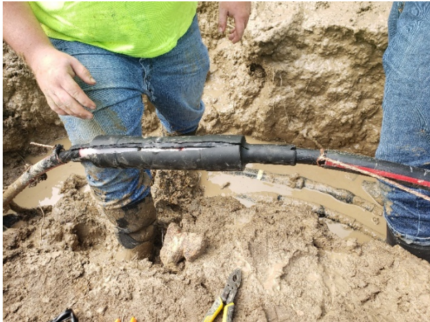
T-10 to T-11 Cable Repair
