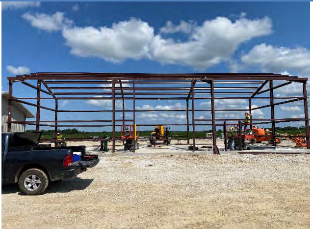
Framing O&M Storage Building
