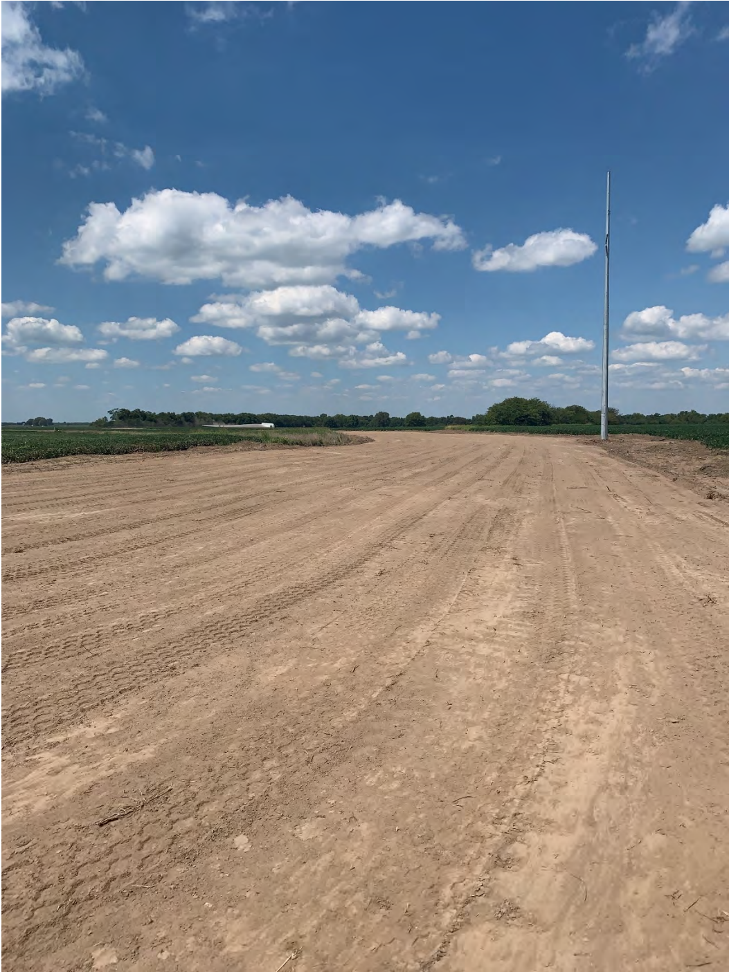
PHOTO 2: CRANE PATH TO T52
