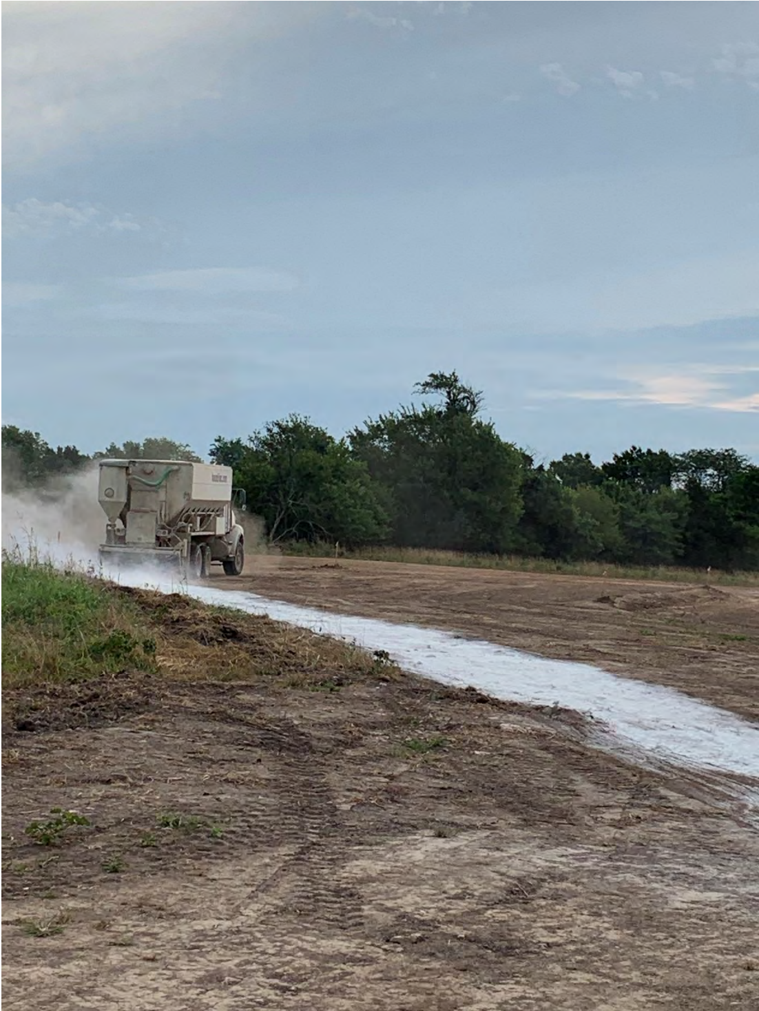
PHOTO 5: H1 PAD STABILIZATION
