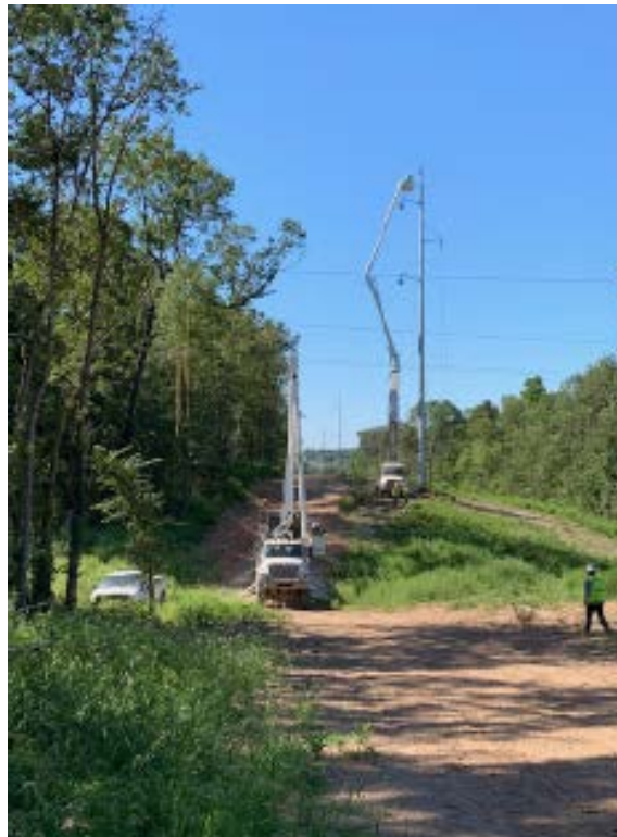
Picture 2. Line construction crews working on generation tie line.
