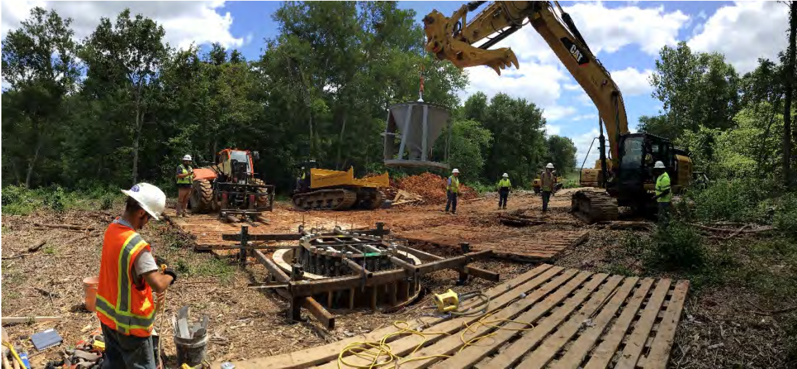
PHOTO 4: T-LINE FOUNDATION
