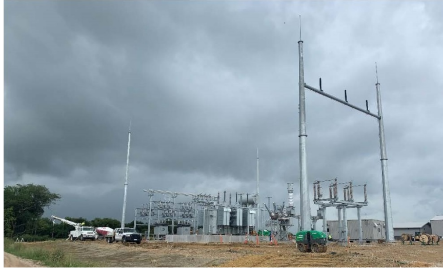
Picture 3. Substation progress as of August 27 th .
