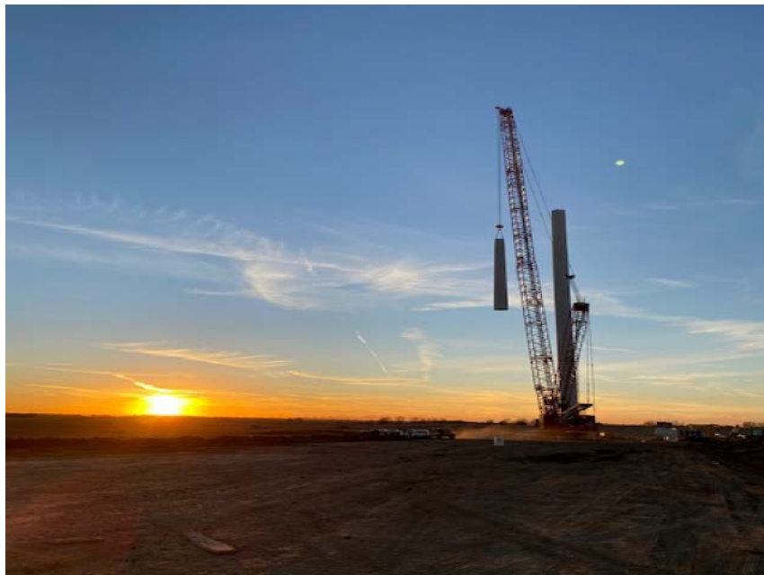
Picture 2. Turbine erection at sunset.
