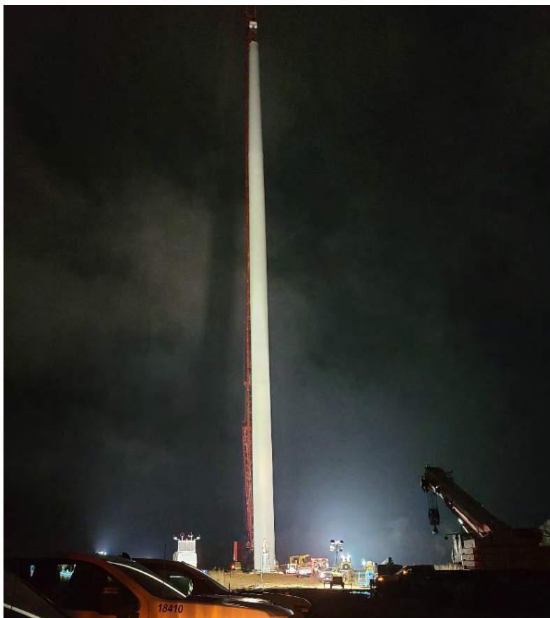
T-52 Night Erection Crew
