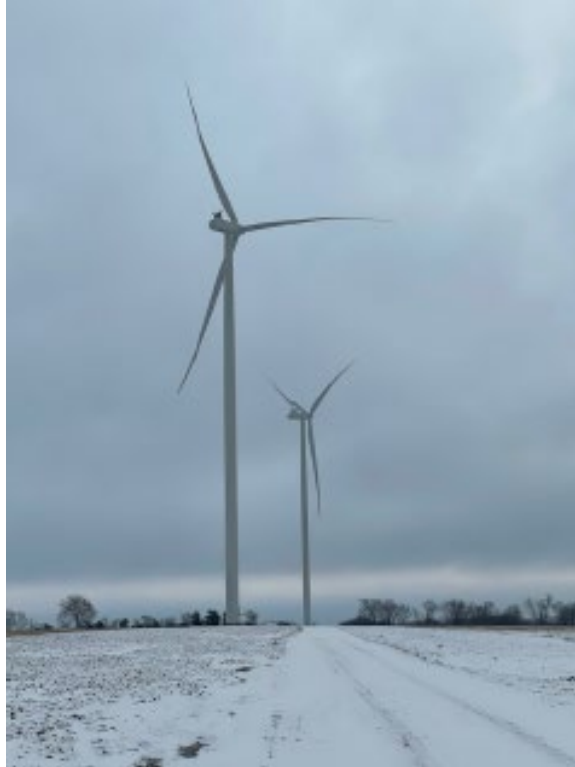
Picture 3. Site activities were again impacted by wintery weather.
