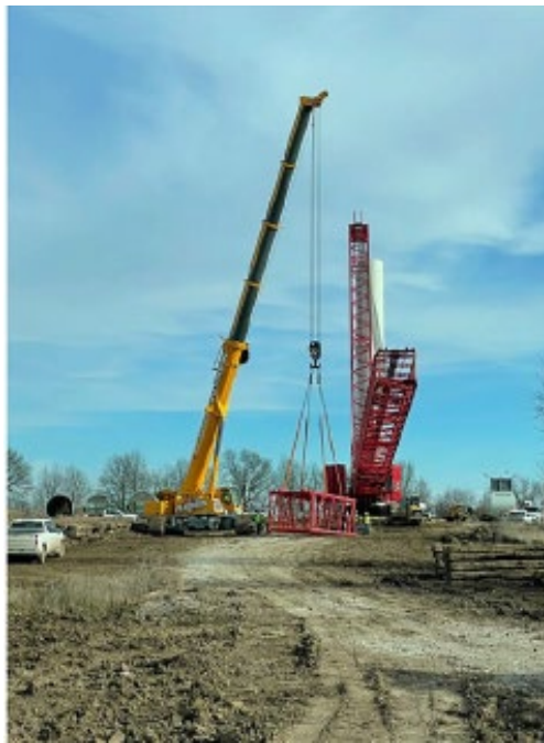
Picture 2. Crane assembly following a breakdown and move.
