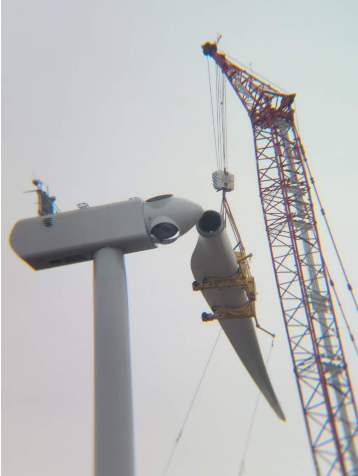
PHOTO 4: T72 BLADE ERECTION
