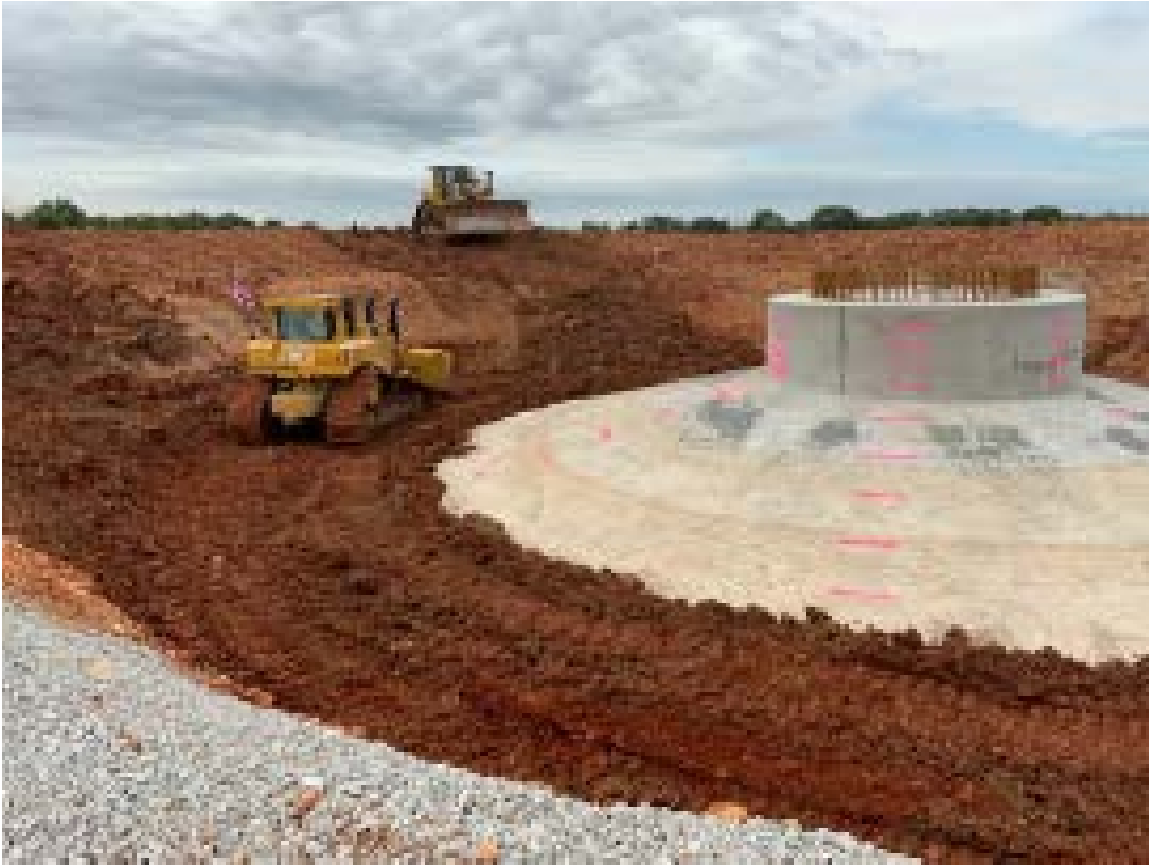
Picture 3. Backfilling a completed foundation.
