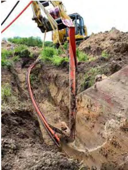
Figure 7.3: Plowing Trench near T30
