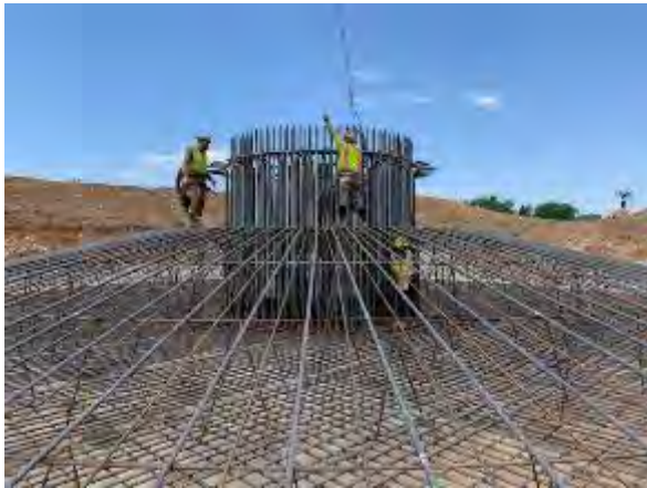
Figure 5.7: T-91 Rebar Cage
