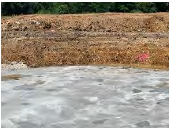
Figure 5.3: T19 Excavation Wall Step Back
