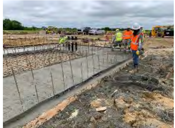
Figure 8.2: Beginning of MPT Foundation
