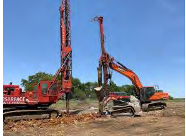
Figure 5.2: T134 Stone Column Installation
