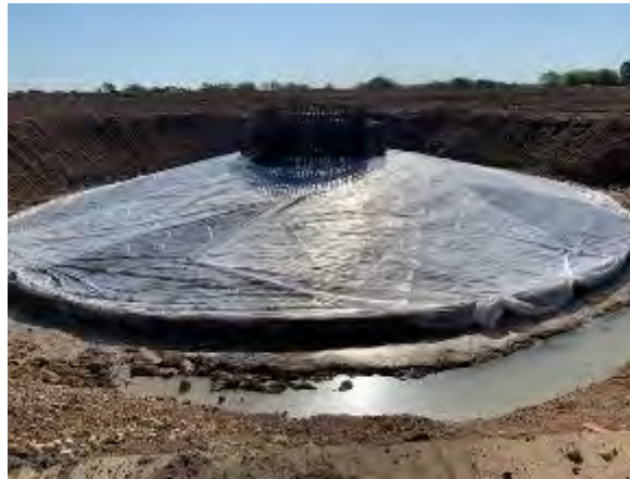
Figure 5.11: Foundation Concrete Curing
