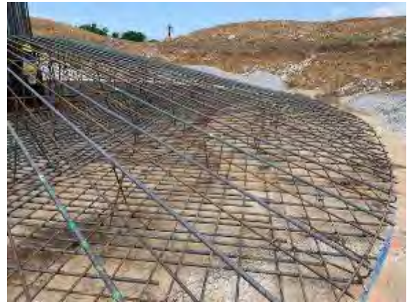
Figure 5.8: T-91 Rebar Cage
