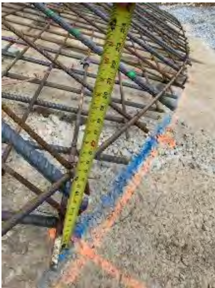
Figure 5.9: Edge of Rebar
