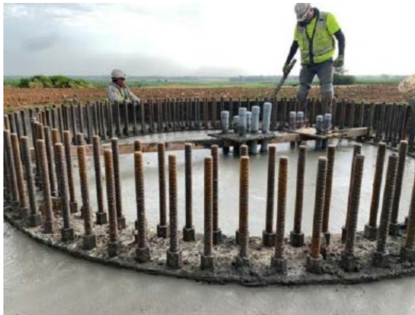
Picture 2. Finishing T-124 foundation pedestal.
