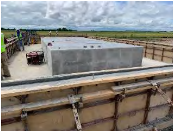
Figure 8.3: Poured MPT Foundation
