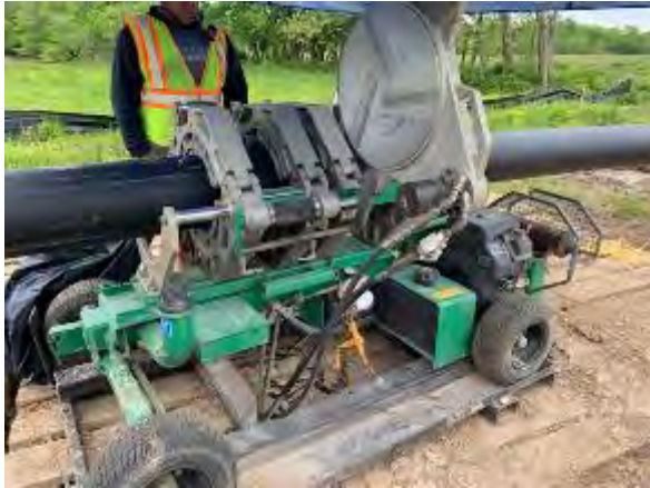
Figure 7.1: Boring Pipe Fusing Equipment
