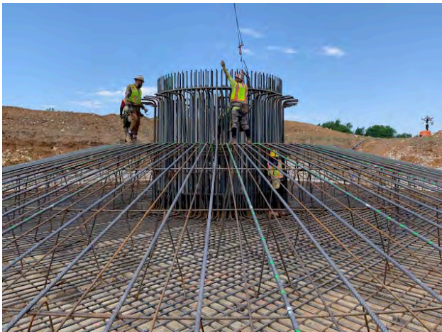
Top Mat Install
