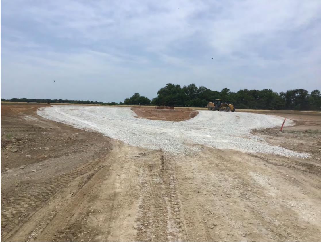
PHOTO 4: T52 H1 PAD
