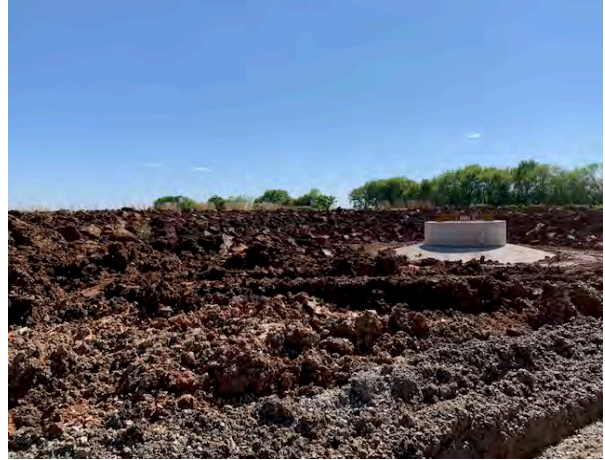
T-55 Foundation backfill
