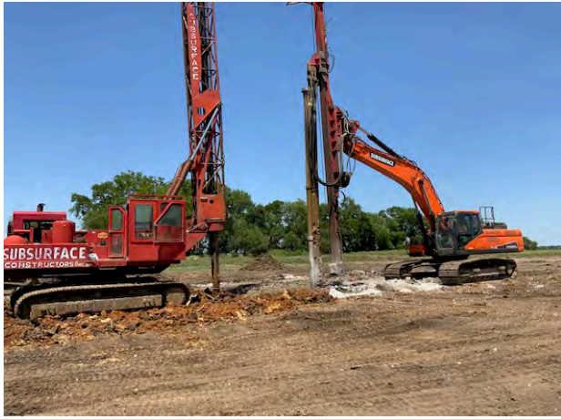
Stone Column Install
