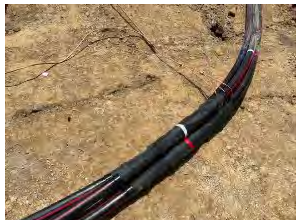
Figure 7.6: T50 Splice
