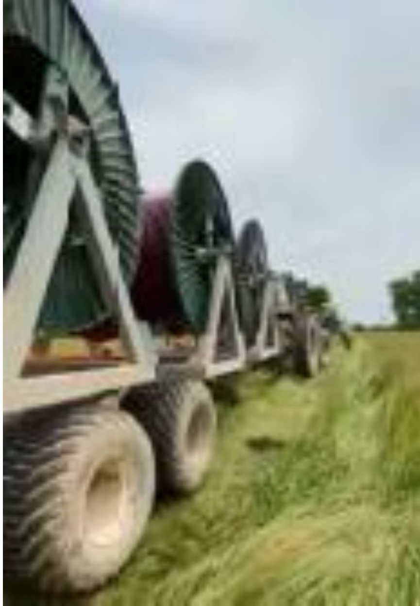
Picture 3. Spider plow loaded with three spools (one for each phase) of collection cable.
