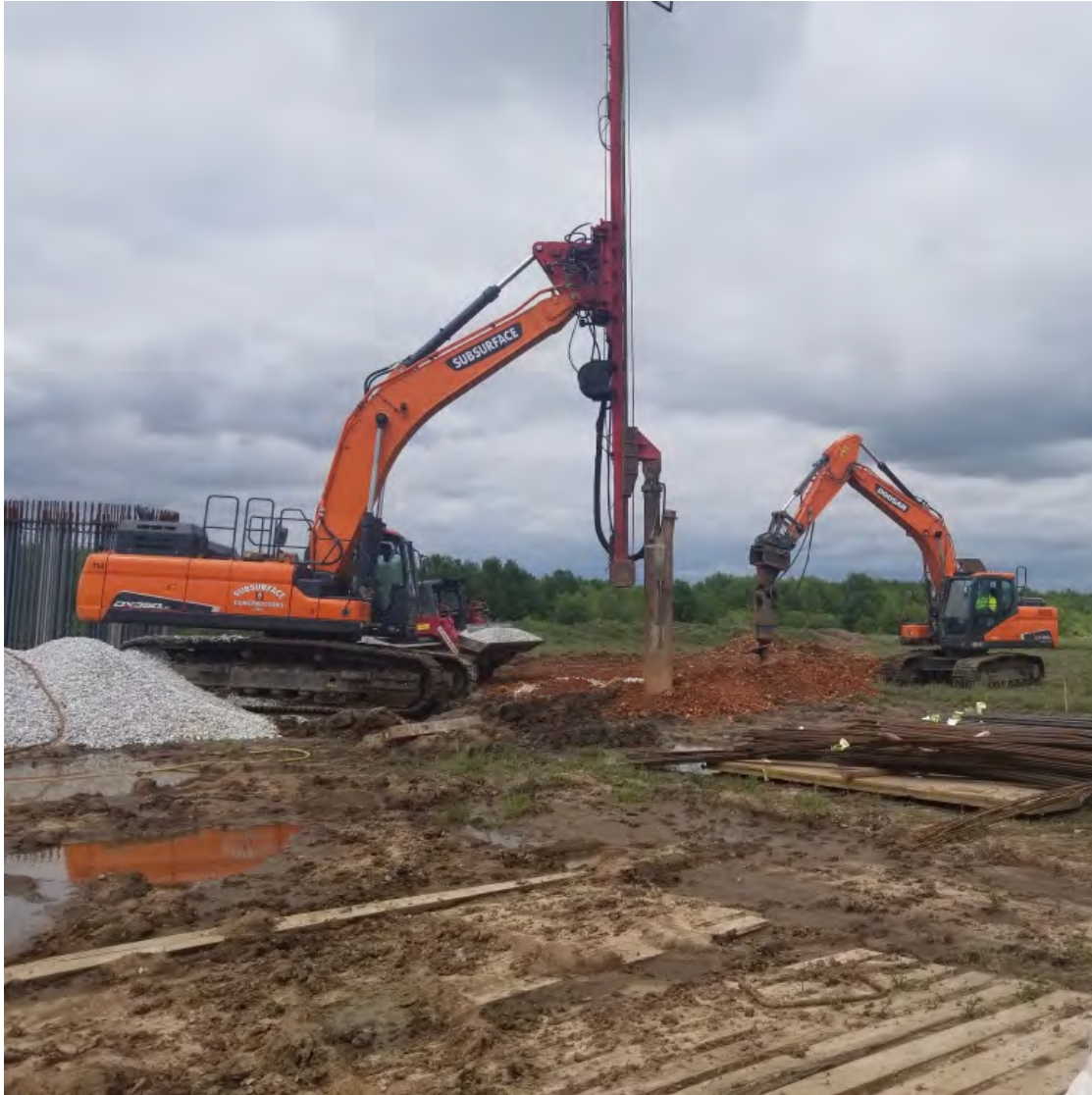
PHOTO 4: STONE COLUMN INSTALLATION
