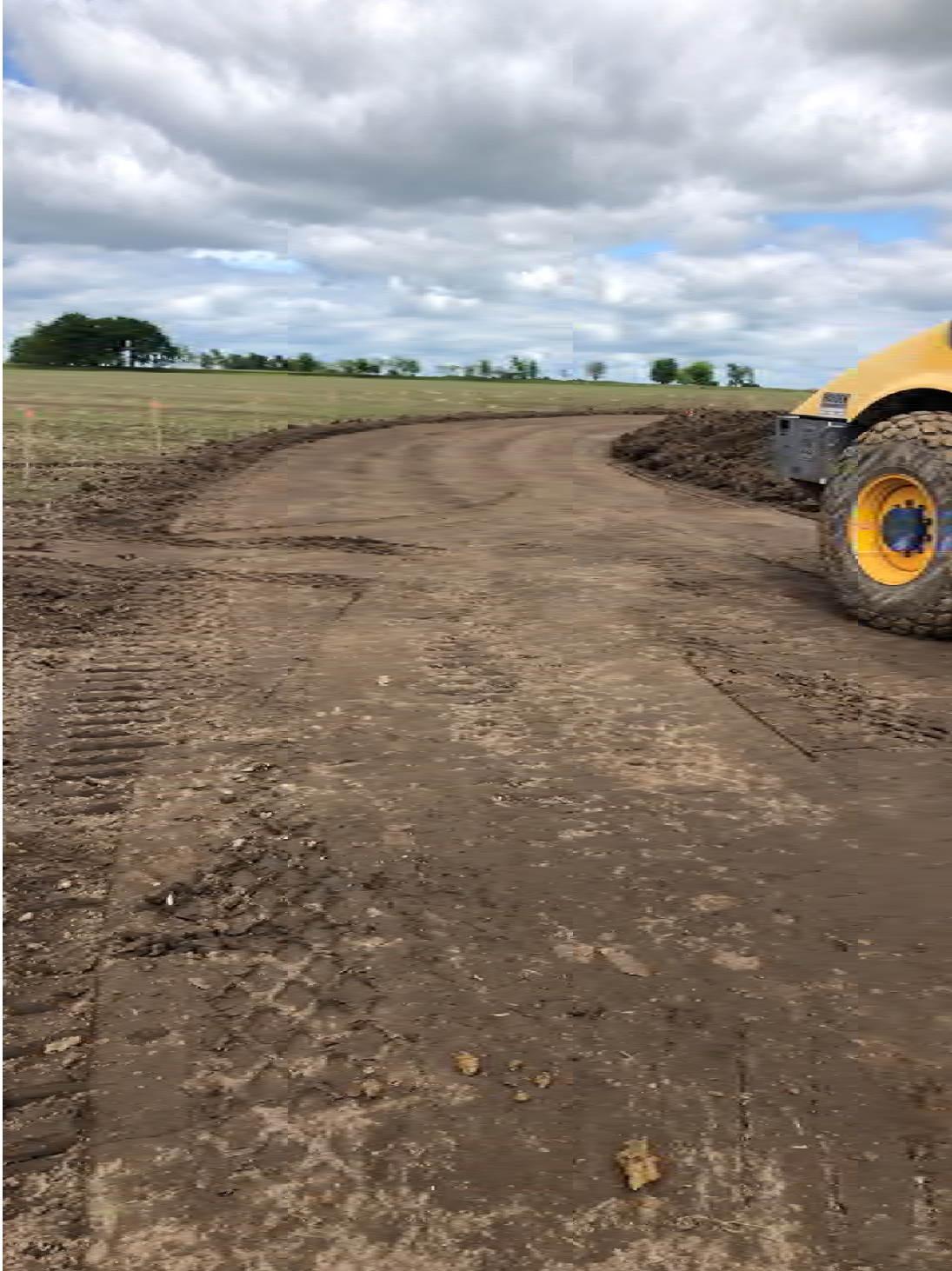
PHOTO 7: PUBLIC ROAD RADII INSTALLATION
