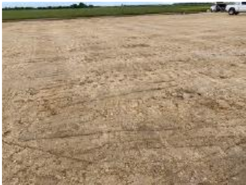
Picture 2. Finished substation pad, ready for foundation installation.
