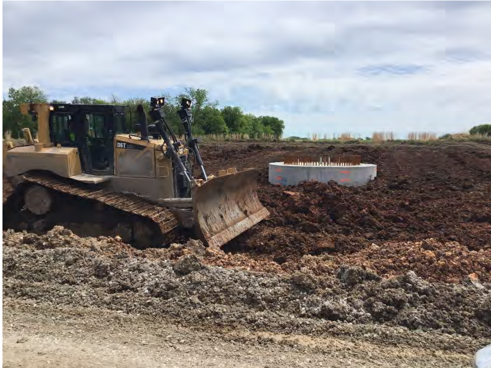
PHOTO 5 & 6: FOUNDATION BACKFILL
