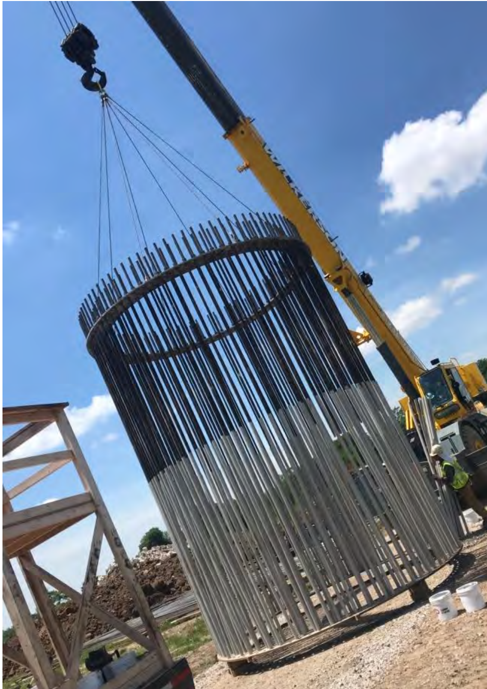
PHOTO 1: AB CAGE BUILD
