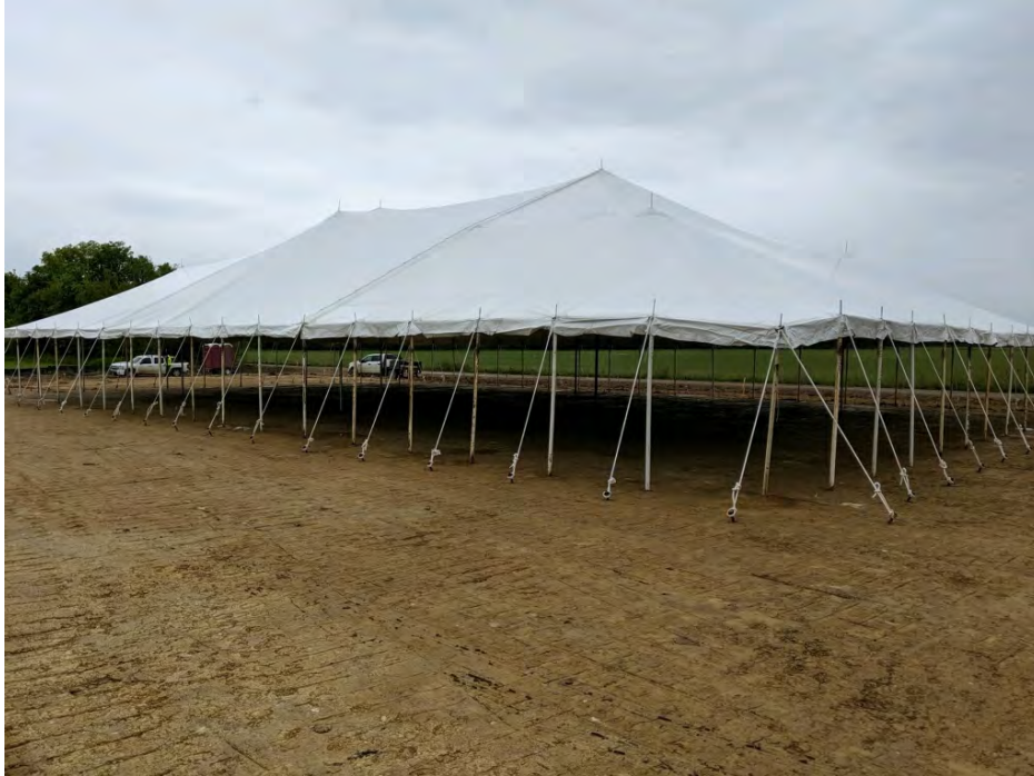
PHOTO 2 & 3: MPT FOUNDATION PREP
