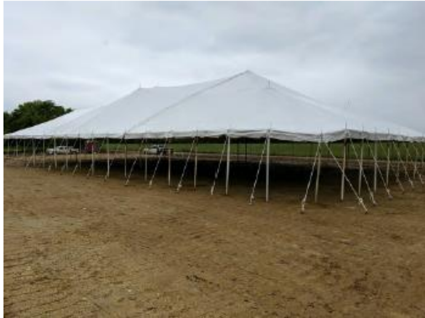
Picture 1. Extreme precipitation amounts required an unusual solution to prepare the transformer pad for delivery of the transformer on schedule.
