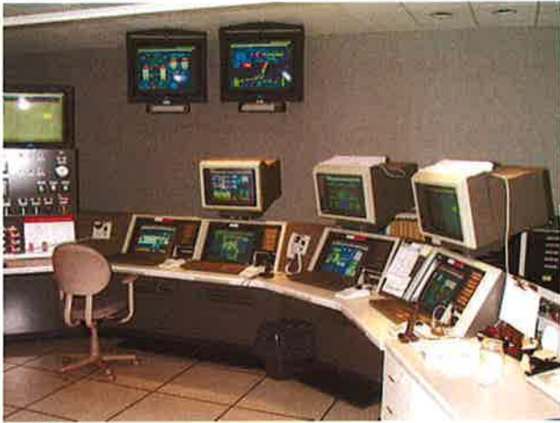
Control Room Remodeling: (Units 1, 2, 3, & 4)
