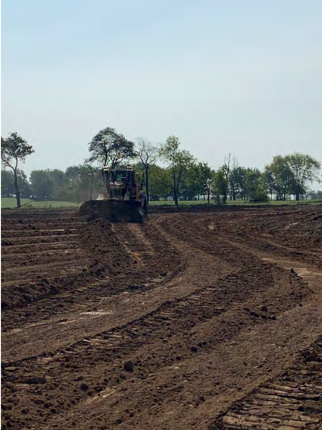
PHOTO 8: CRANE PATH GRADING
