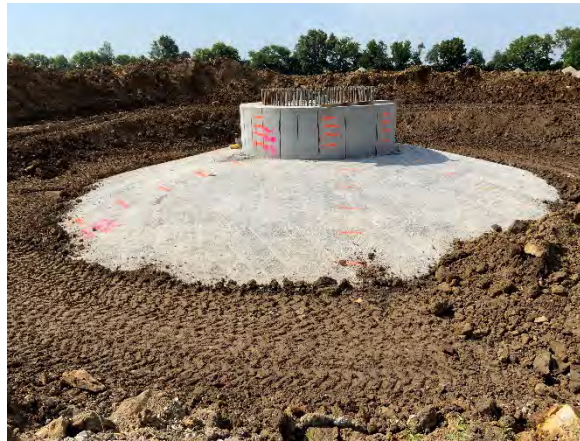
Figure 5.1: T133 Backfill in Progress
