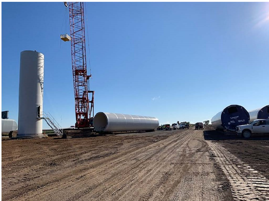
Picture 2. Mid-tower sections staged and awaiting erection.
