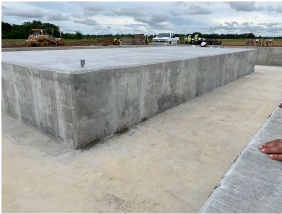
Figure 7.7: Substation MPT Foundation
