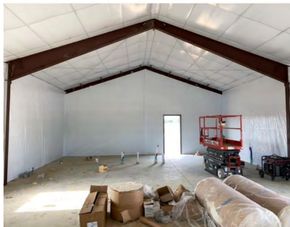
Figure 10.3: O&M Building Interior
