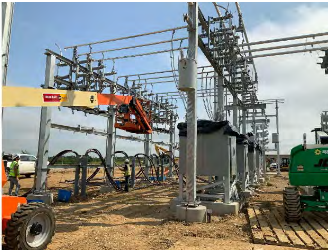
Installing Jumpers
