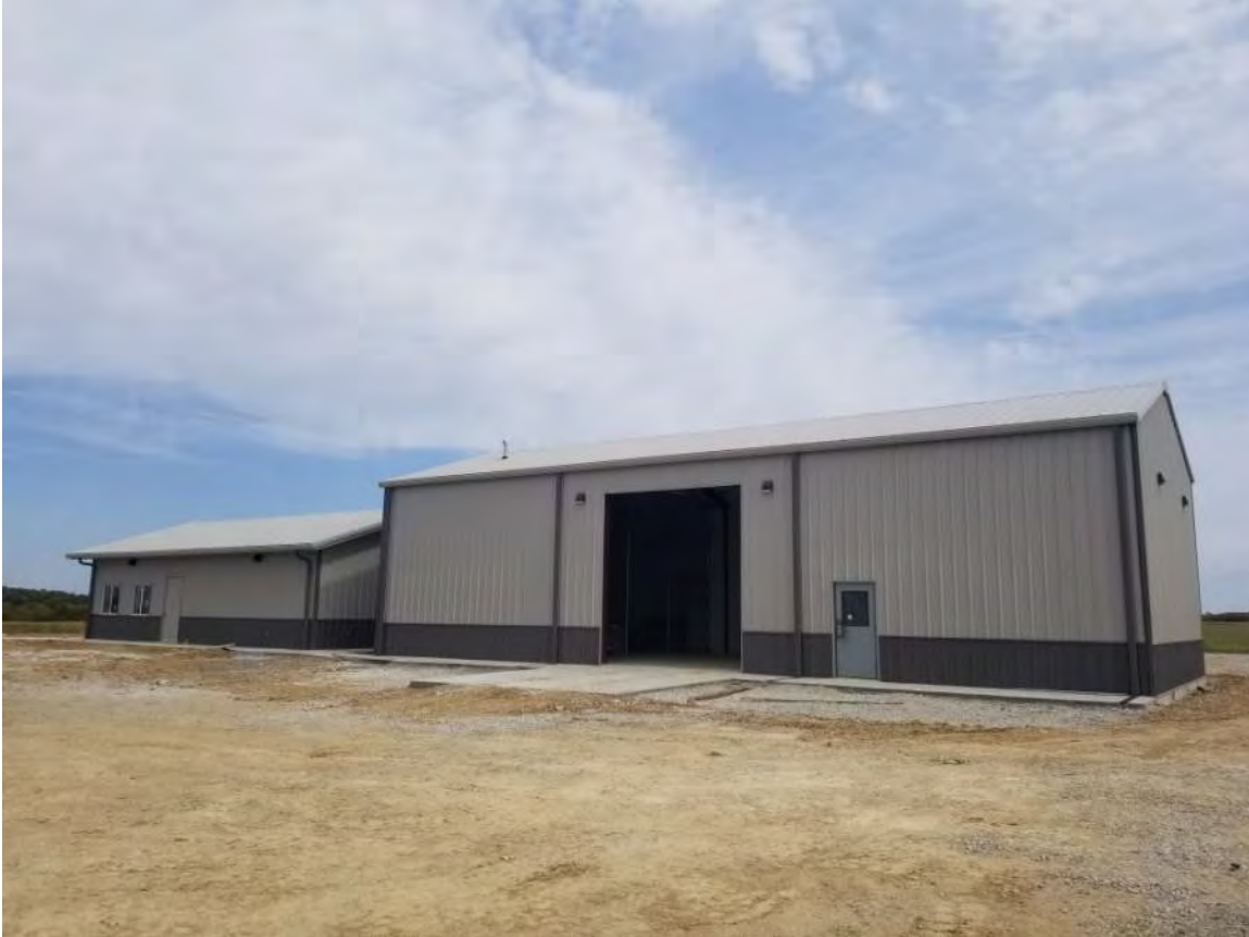
PHOTO 5: O&M AND STORAGE BUILDING
