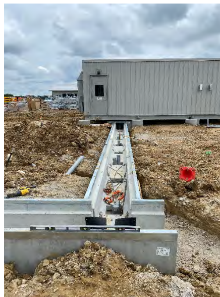
Figure 7.7: Installation of Trenwa
