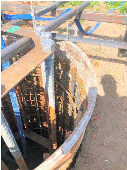
Figure 9.3: T-Line Structure Foundation Form
