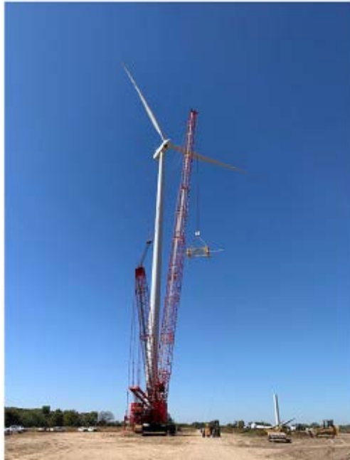
Picture 1. Lifting a blade into place to top out a turbine.
