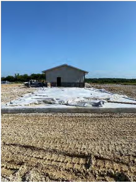
Figure 10.1: O&M Building Exterior and Additional Storage Building Pad
