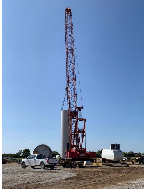
Picture 3. Placing a base tower section.
