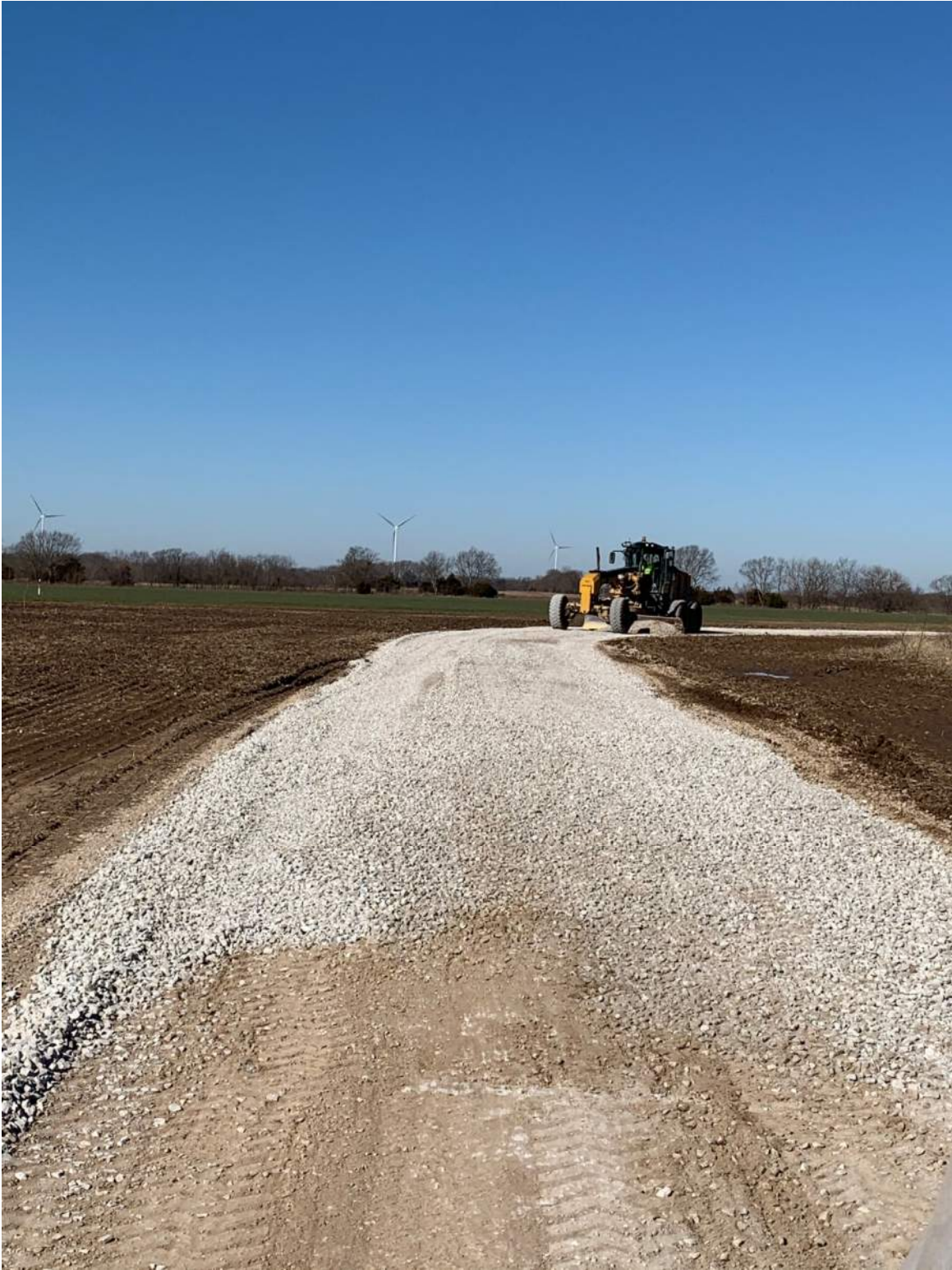
PHOTO 3: 2IN ACCESS ROAD CAP INSTALLATION
