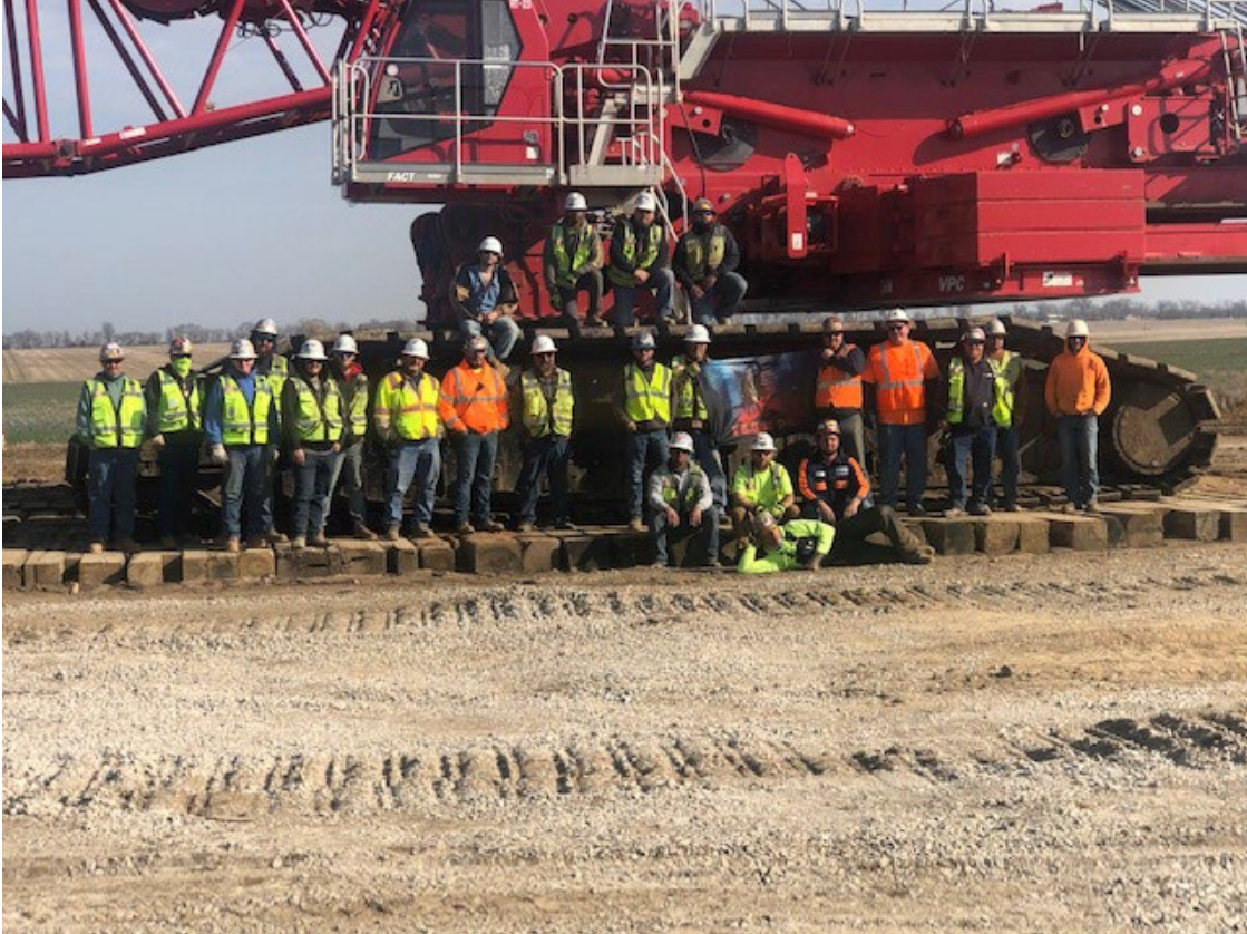
Picture 2. A crew photo to commemorate the completion of turbine erection.
