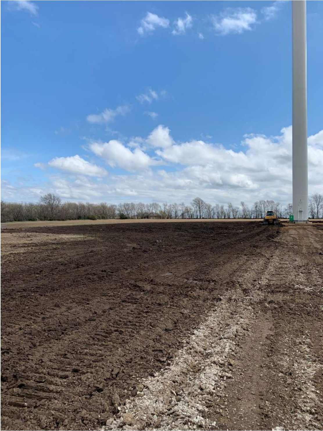
PHOTO 4: T63 SITE RECLAMATION
