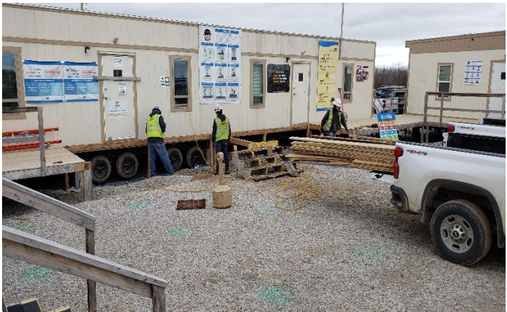
Safety Trailer Demobilization
