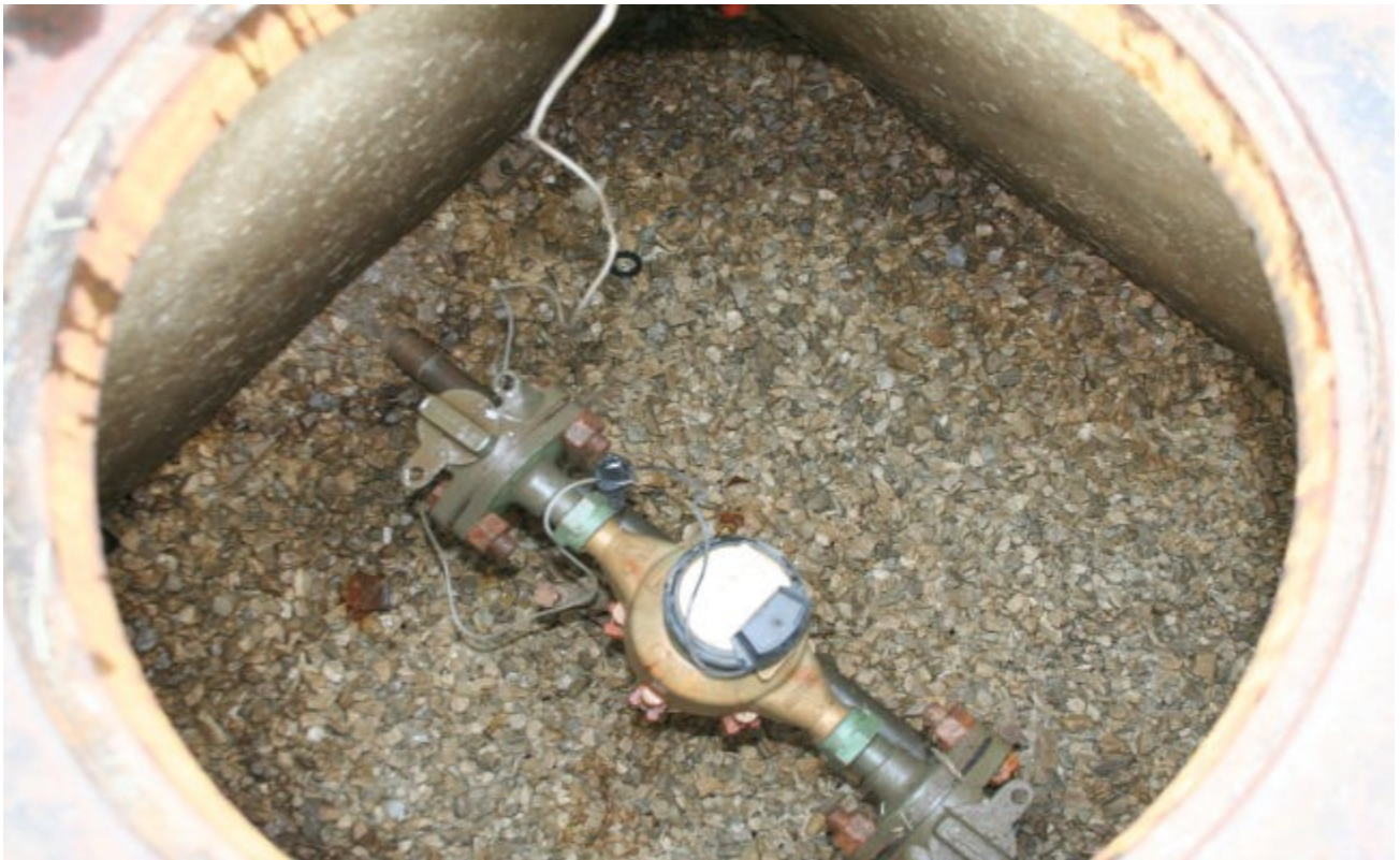
Above picture shows no water in water meeter housing one day latter on July 22, 2009.
