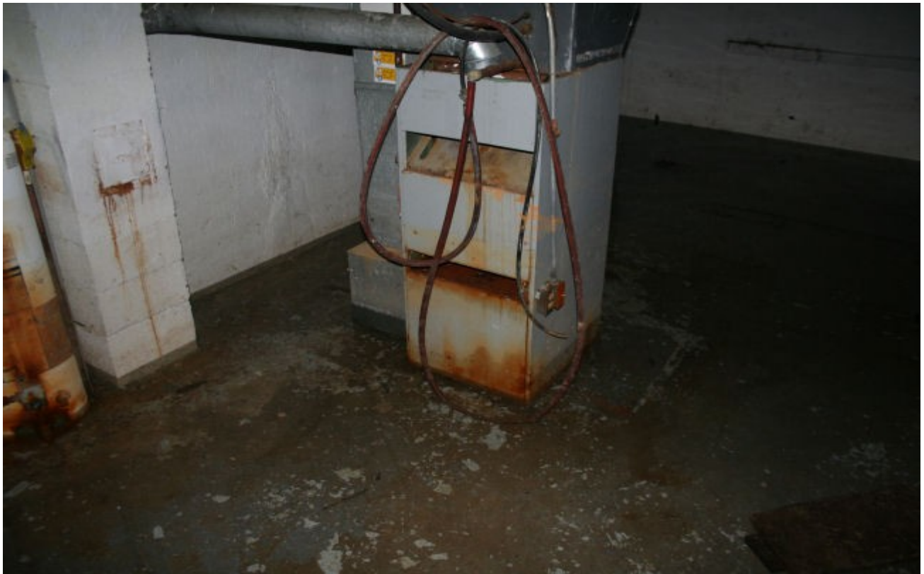
Notice the water marks on the walls and the hot water heater.
