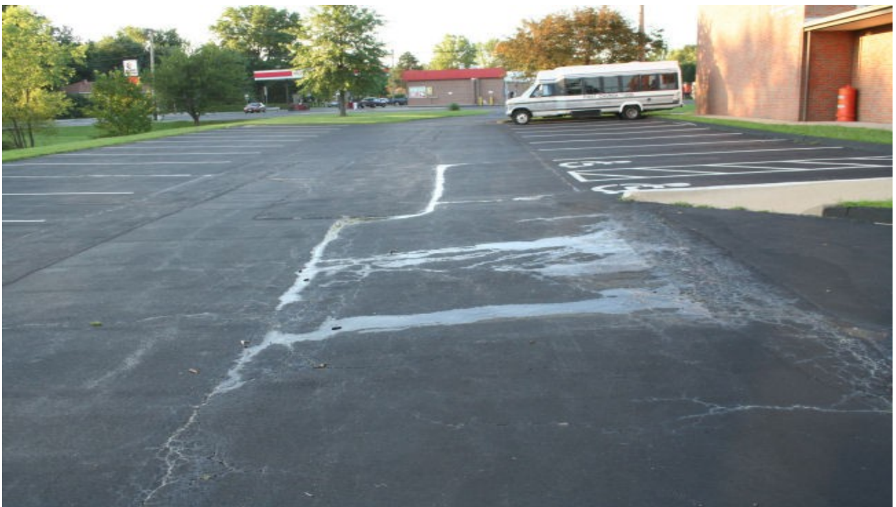
July 13, 2009 Water seeping out of cracks causing damage in west parking lot at the First Church of God parking lot.
