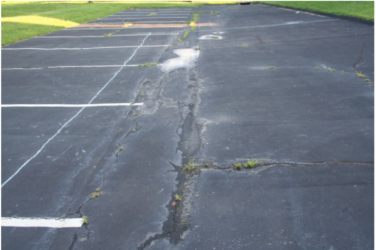
Above two photos: July 13, 2009 Water seeping out of cracks causing damage in east parking lot at the First Church of God parking lot.
