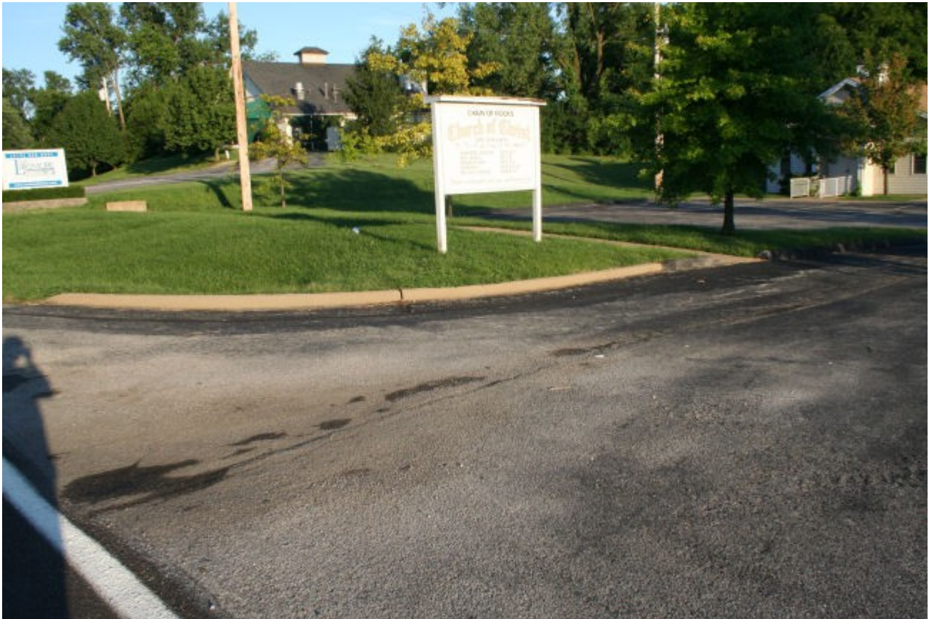
July 13, 2009 Water seeping out of cracks causing damage in parking lot at Chain of Rocks Church of Christ 1136 Coal Bank Rd
