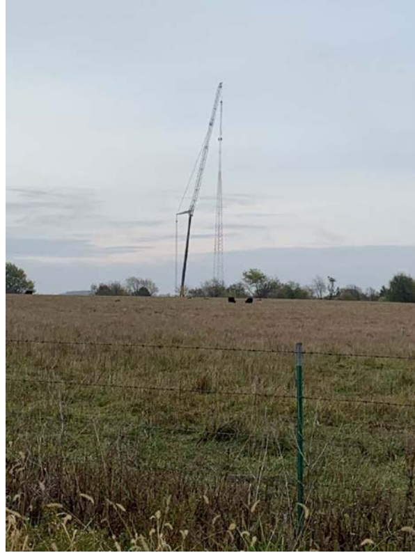
Picture 3. Permanent met tower erection.
