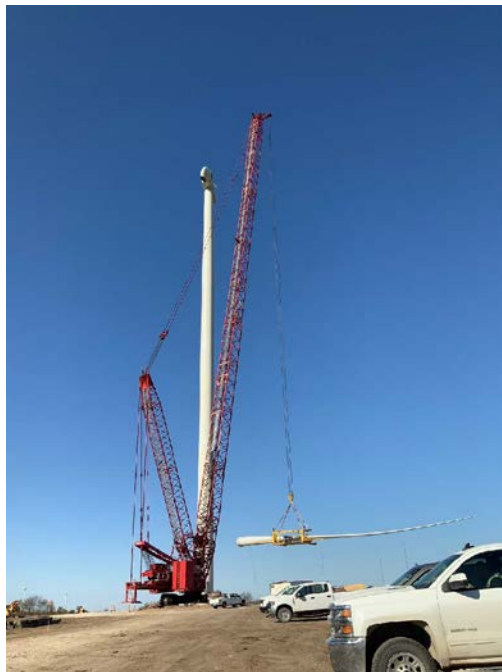
Picture 2. Lifting a turbine blade to complete top out.
