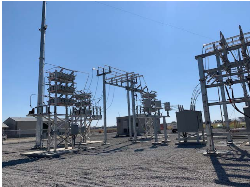
Picture 1. Substation progress on October 8 th , 2020.
