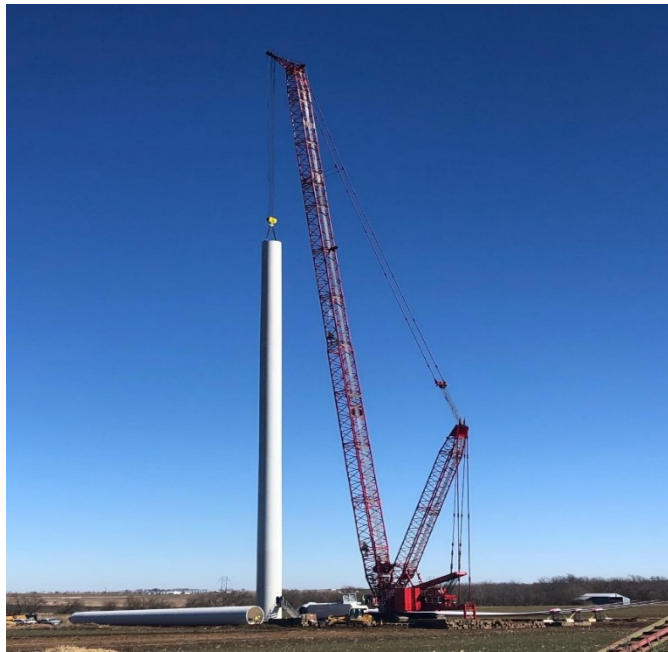
Picture 1. Main erection at T-20.
