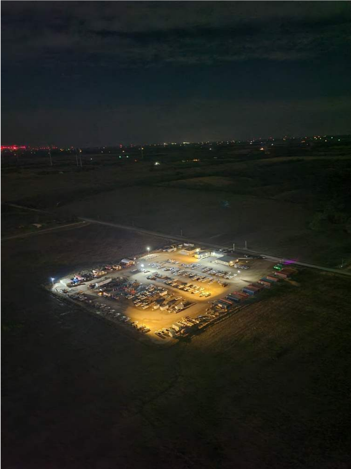
PHOTO 5: LAYDOWN YARD AT NIGHT
