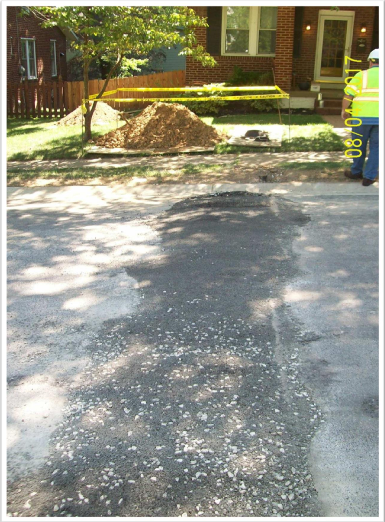
An example of a LSL replacement where the water main is on the opposite side of the street from the customer's home. This photograph is in the St. Louis County service area where the customer owns the entire service line.
