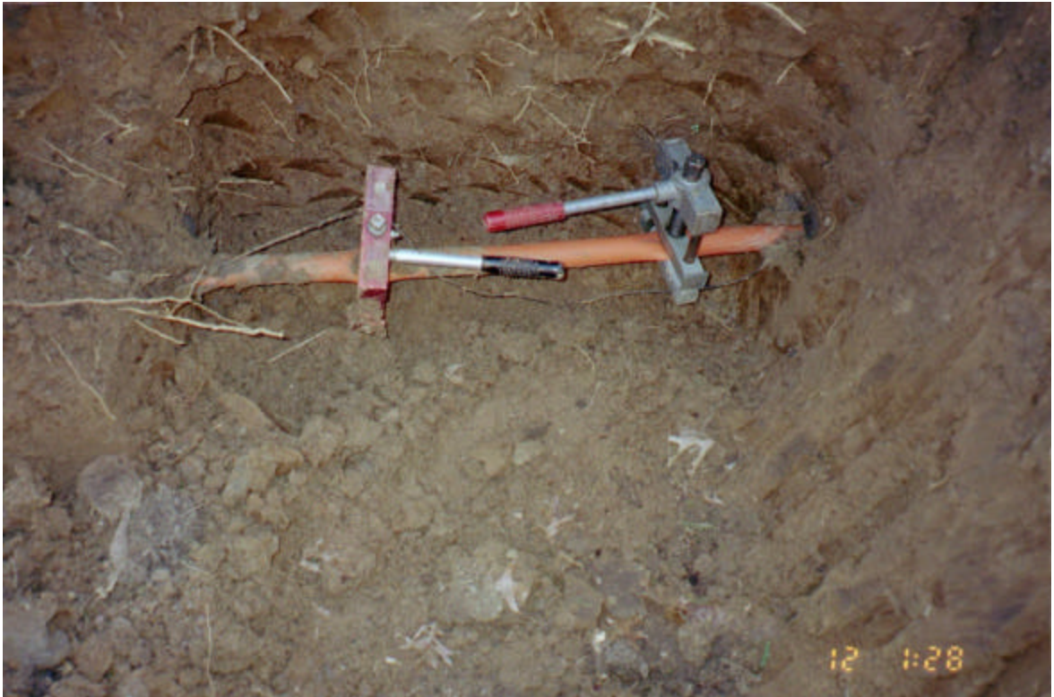
Photograph 3 Squeeze-off of distribution main near #14 Hagers Mill Court.
