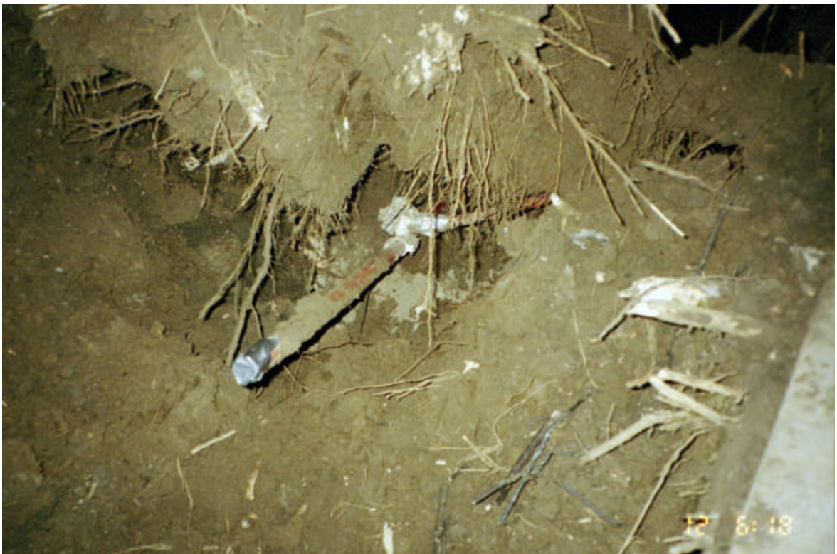
Photograph 12 Tree root ball being lifted from ground. Section of distribution main, service tee and service line are suspended by the tracer wire. Dry soil can be seen beneath the service tee.
