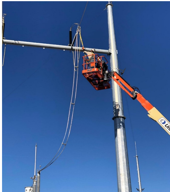
Picture 1. Removing generation tie line grounds prior to energization.
