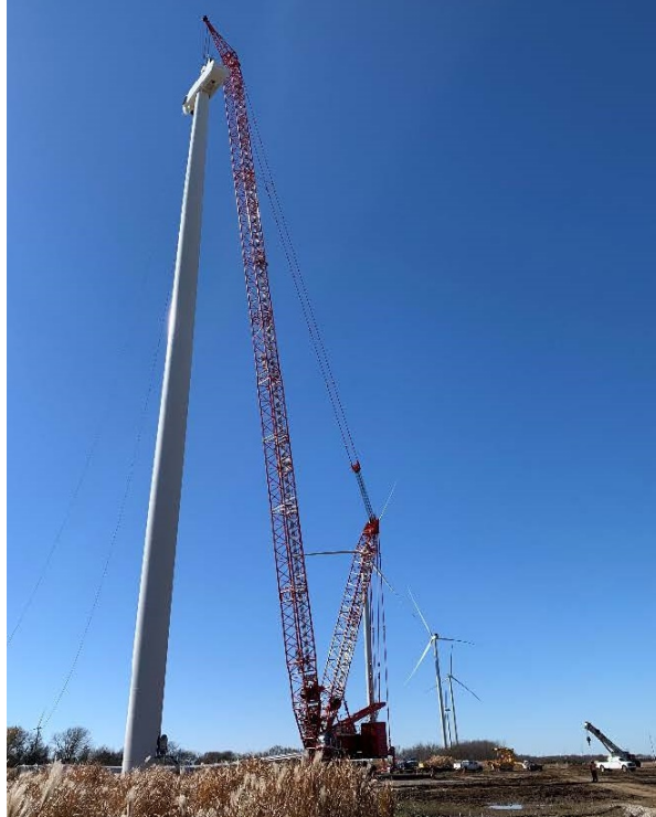
Picture 3. Setting a turbine nacelle to commence top out.
