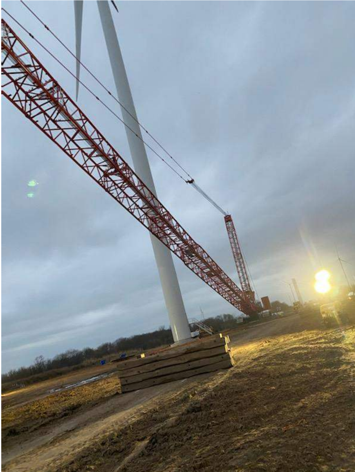
PHOTO 2: ME CRANE BREAKDOWN
