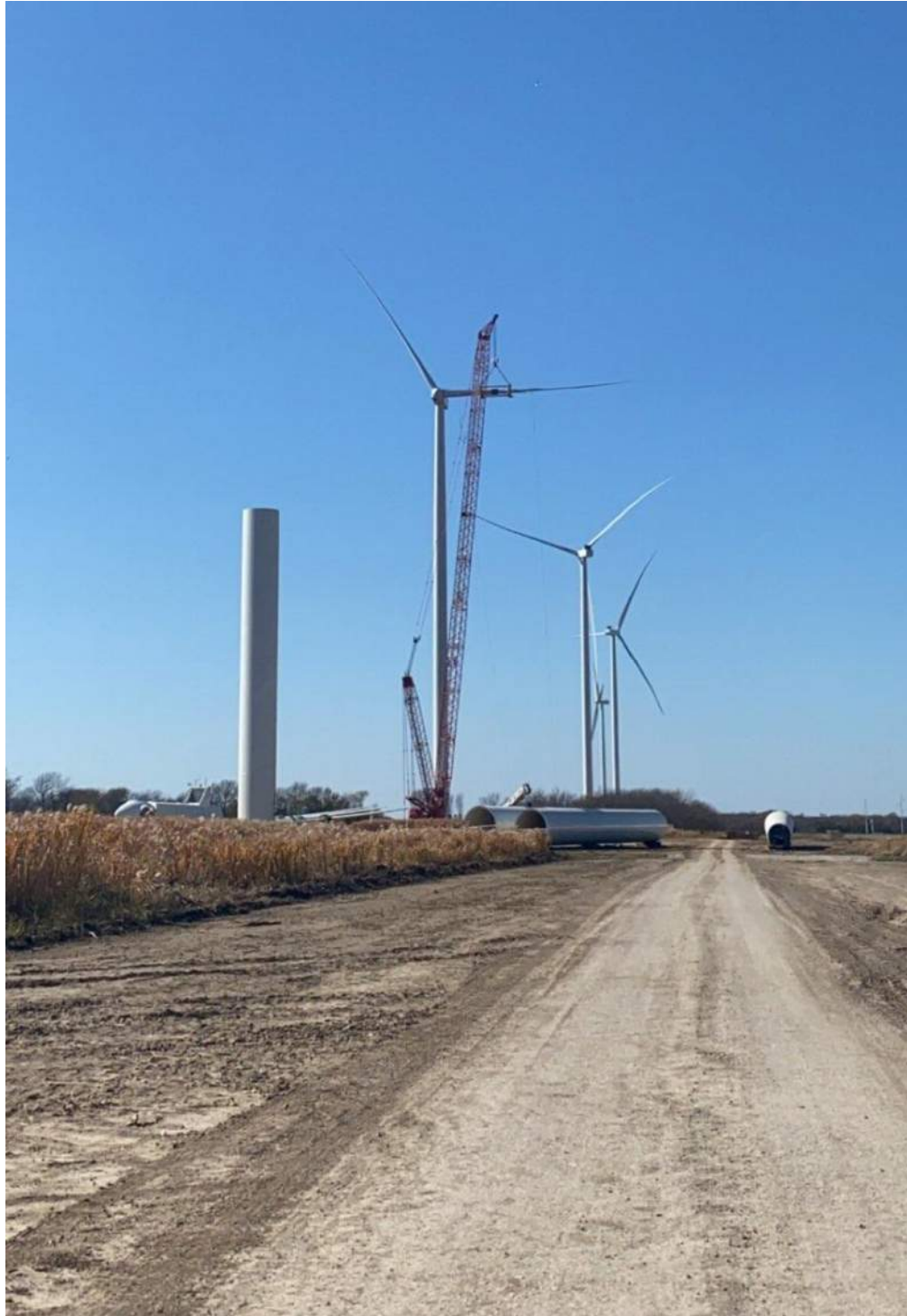
PHOTO 4: MAIN ERECTION - BLADES
