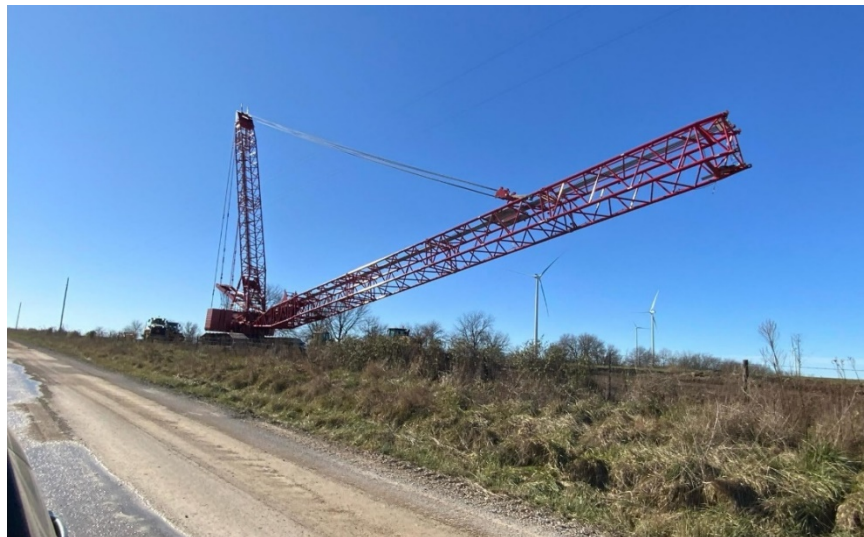
Picture 2. Crane walking to the next turbine site.
