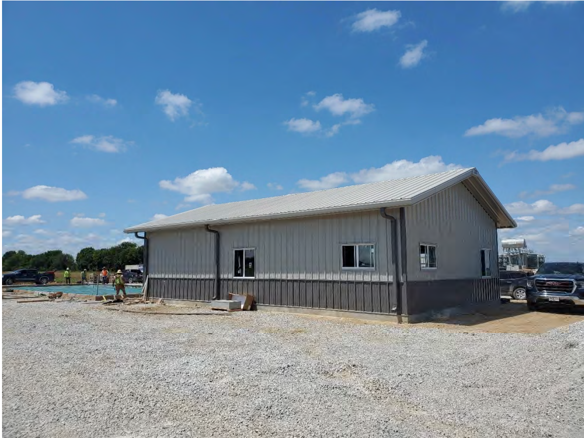
PHOTO 6: O&M BUILDING, STORAGE BUILDING FOUNDATION PREP
