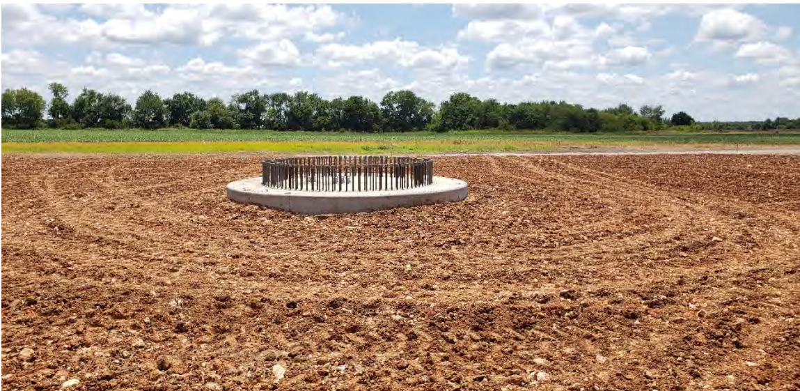
PHOTO 2: WTG FOUNDATION BACKFILL COMPLETE
