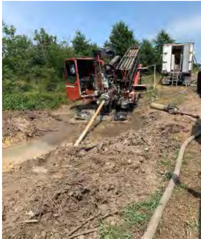
Picture 1. Directional boring for collection system.
