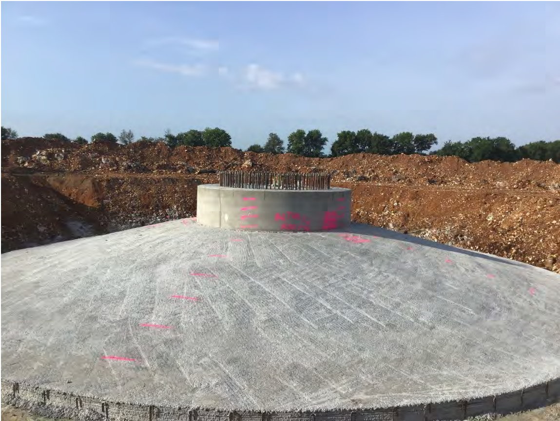
PHOTO 2: WTG FOUNDATION BACKFILL COMPLETE
