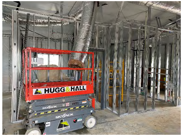
O & M Building Paneling and Interior Framing
