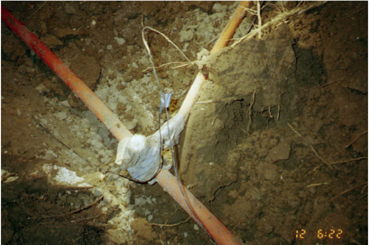
Photograph 13 Distribution main, service tee, service line and tracer wire serving #6 Hagers Mill Court.
