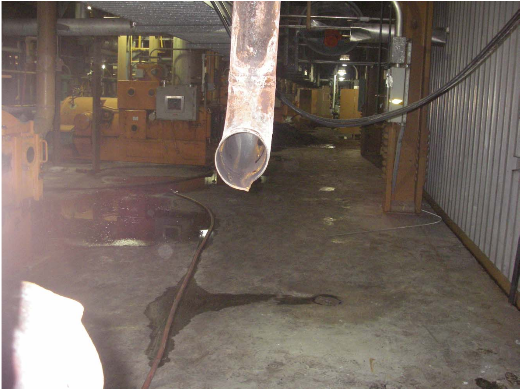
PHOTOGRAPH # 2 VIEW OF DAMAGED PIPE WITH COAL FEEDERS IN BACKGROUND
