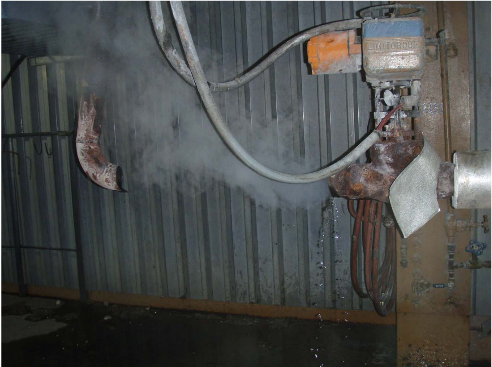
PHOTOGRAPH # 1 LOCATION OF PIPE RUPTURE
