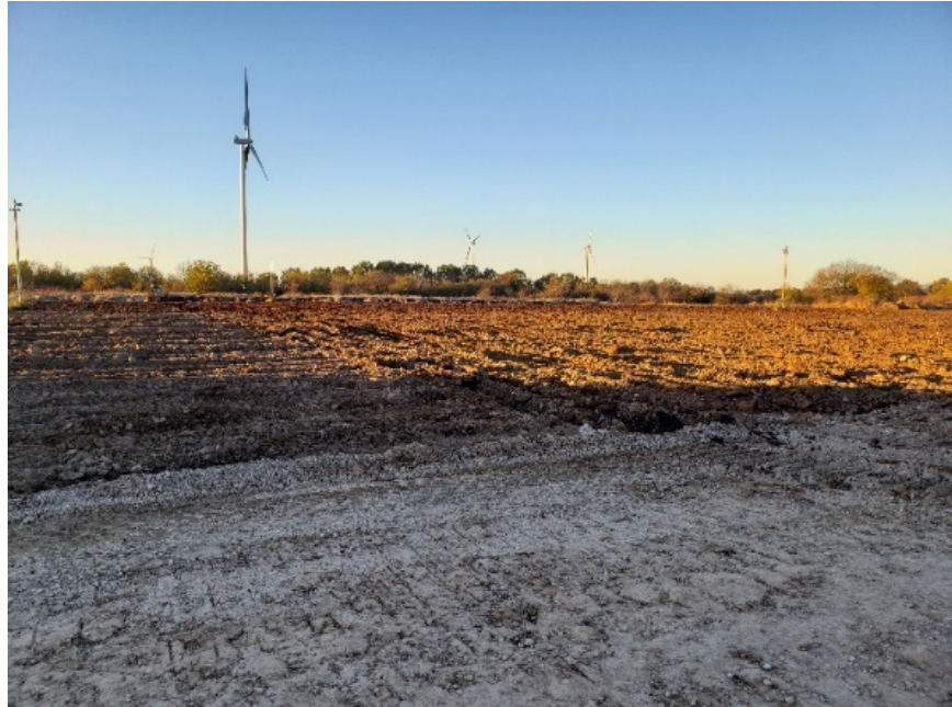
Picture 1. Laydown yard reclamation in progress.
