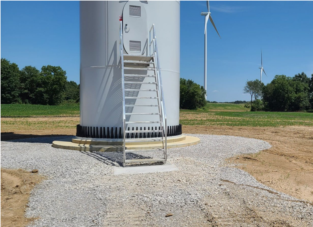
Final Restoration, Turbine Beauty Ring
