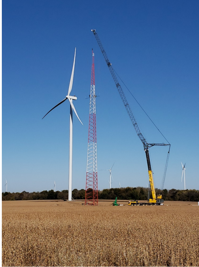
Picture 3. Permanent met tower erection.
