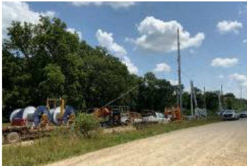
Picture 4. Pulling conductor for the generation tie line.
