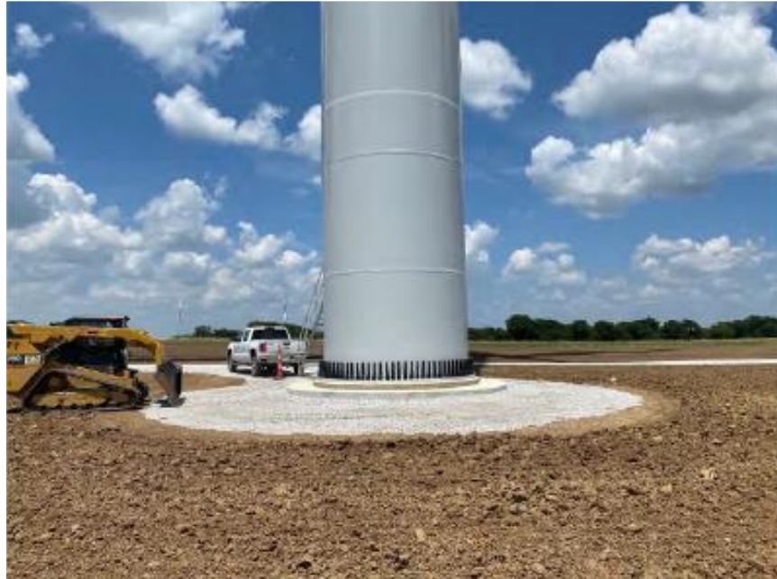
Picture 3. Reclaimed and restored turbine site. The site will be re-vegetated to the landowner's specification.
