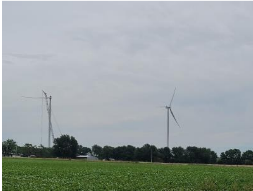
Picture 1. Stabbing blades on to an erected turbine.
