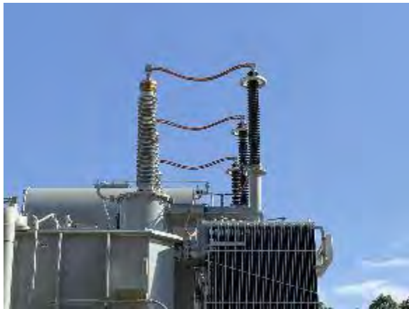
Figure 8.3: MPT HV Bonding Jumper
