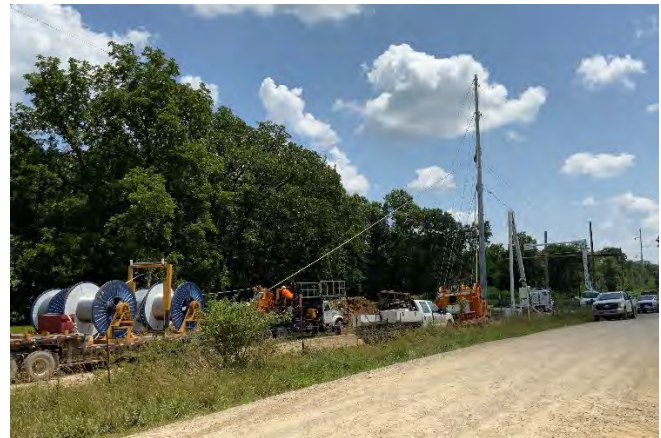
Transmission Line Conductor Pull
