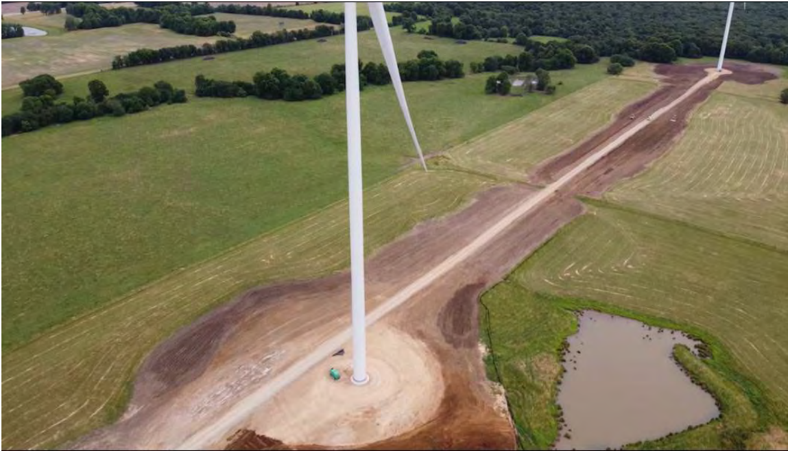
PHOTO 1: RESTORATION AT T-94 & T-99
