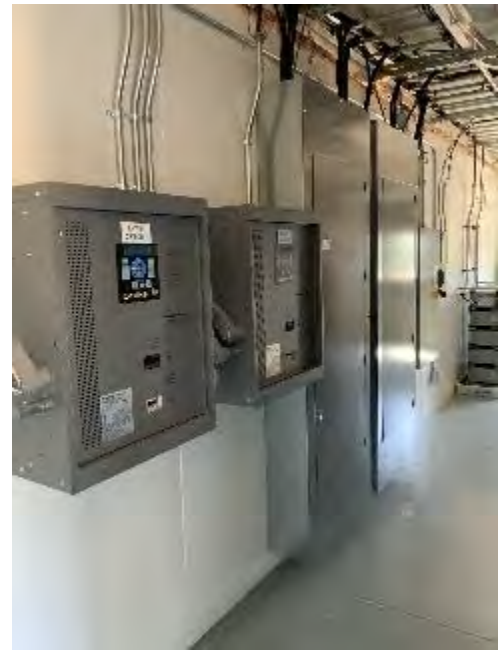
Figure 8.8: Battery Chargers
