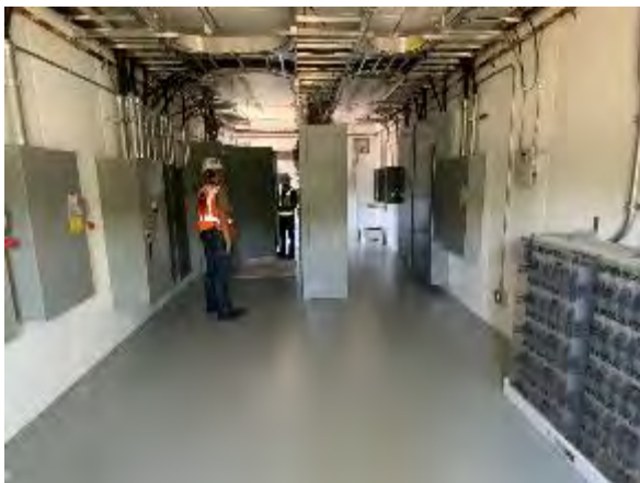
Figure 8.5: Control Building View From Eastern Door
