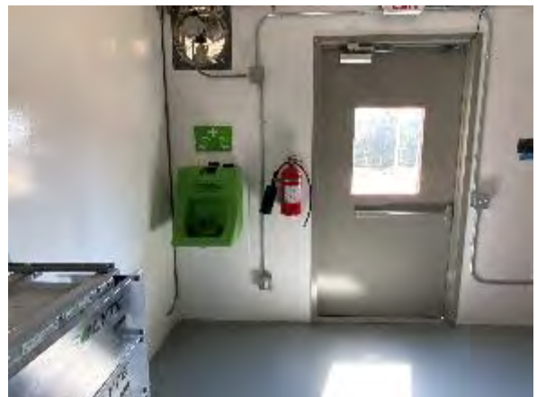
Figure 8.6: Eyewash Station by Eastern Door
