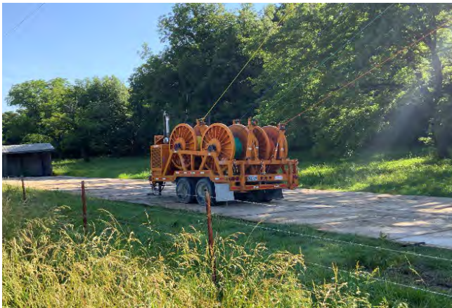
Transmission Line Conductor Pull
