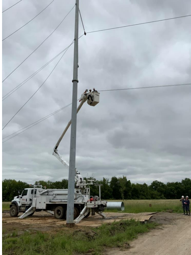
Picture 3. Stringing conductor on the generation tie line.
