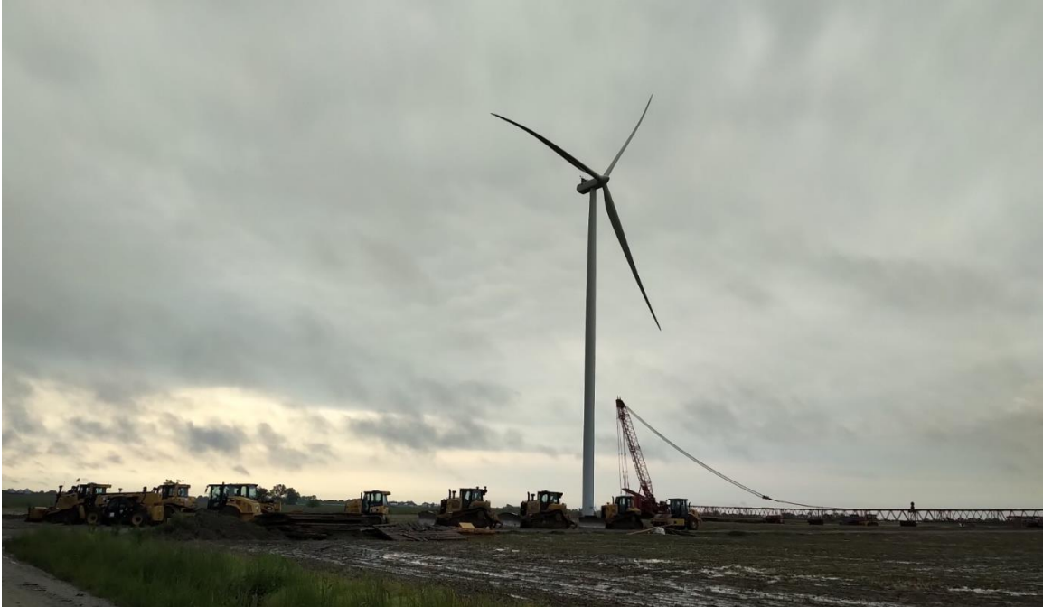
PHOTO 5: T-94 TOP OUT, CRANE BREAKDOWN AND CIVIL SITE PAD PREP EQUIPMENT
