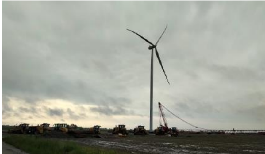
Picture 1. Crane breakdown following top out of T-94.
