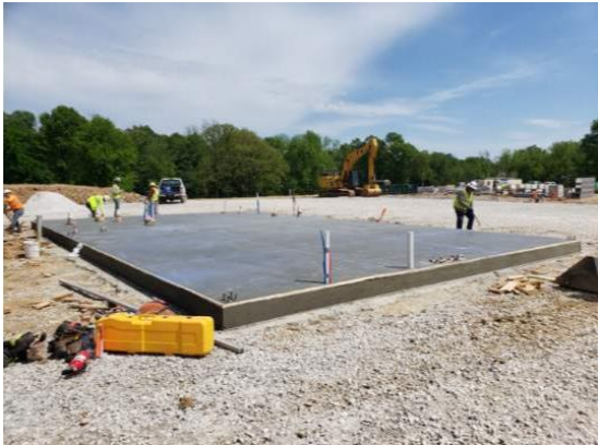
PHOTO 4: O&M BUILDING PROGRESS
