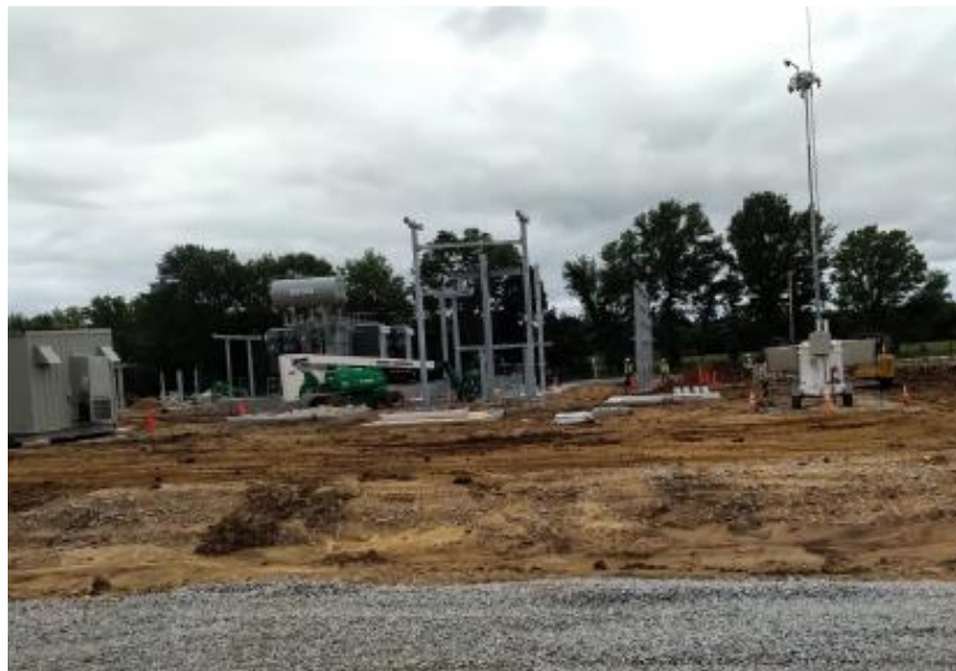
Picture 2. Substation structural steel erection (control building visible at left).
