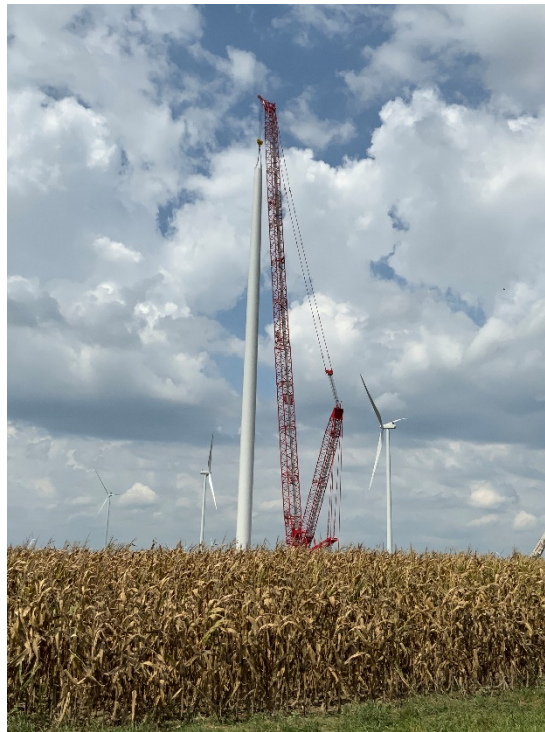
Picture 2. Placing a mid-tower section near the end of main erection activities.
