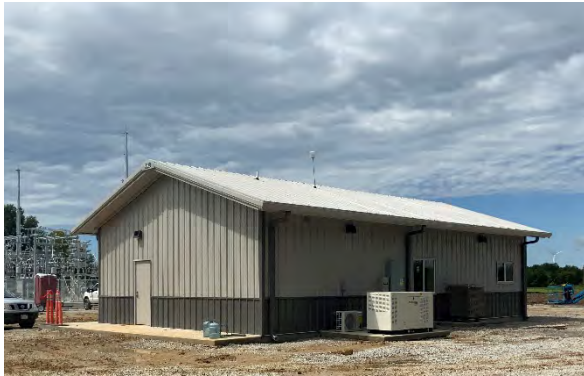
Figure 10.1: O&M Building Exterior
