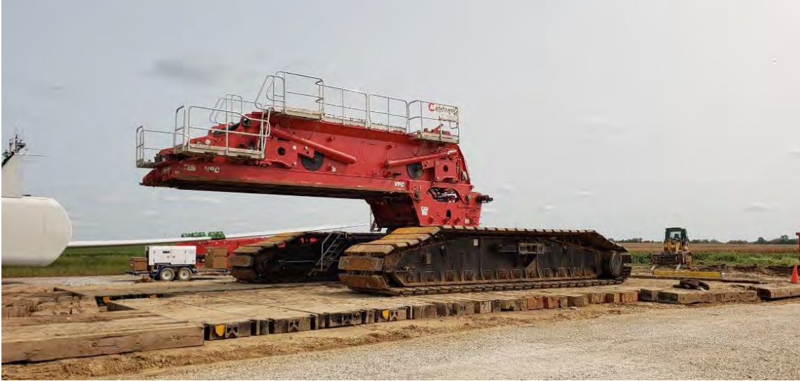
PHOTO 4: LAST 650 LOAD OUT - DEMOB
