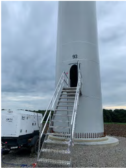
Figure 6.5: T-93 Stairs and Entry Door
