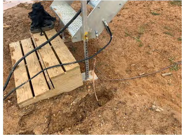
Figure 7.2: Stair Grounding
