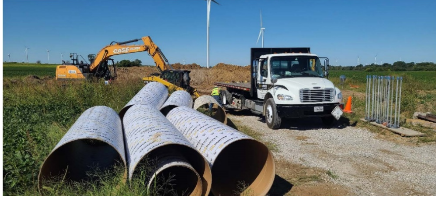
Picture 1. Excavating for permanent met tower foundation.
