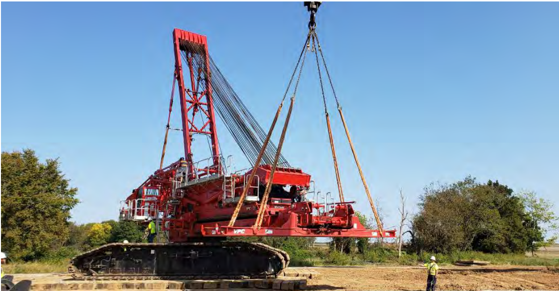
PHOTO 5: LAST 650 LOAD OUT - DEMOB
