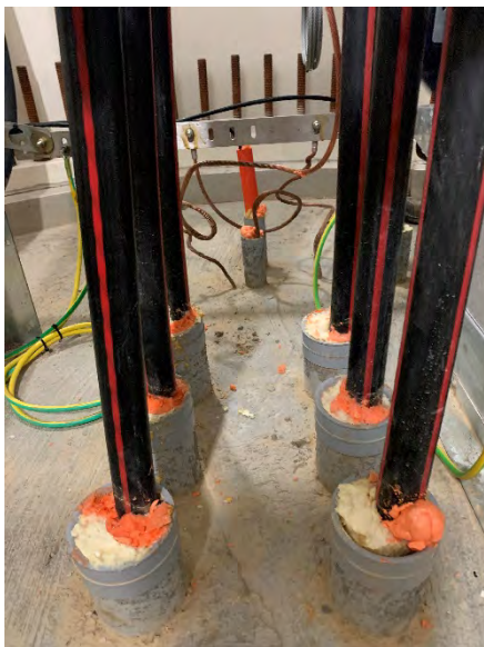
Figure 6.7: Basement Conduits With Foam Filling
