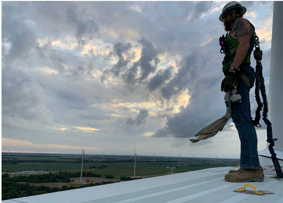
PHOTO 7: WALKDOWN LEAD ON TOP OF NACELLE
