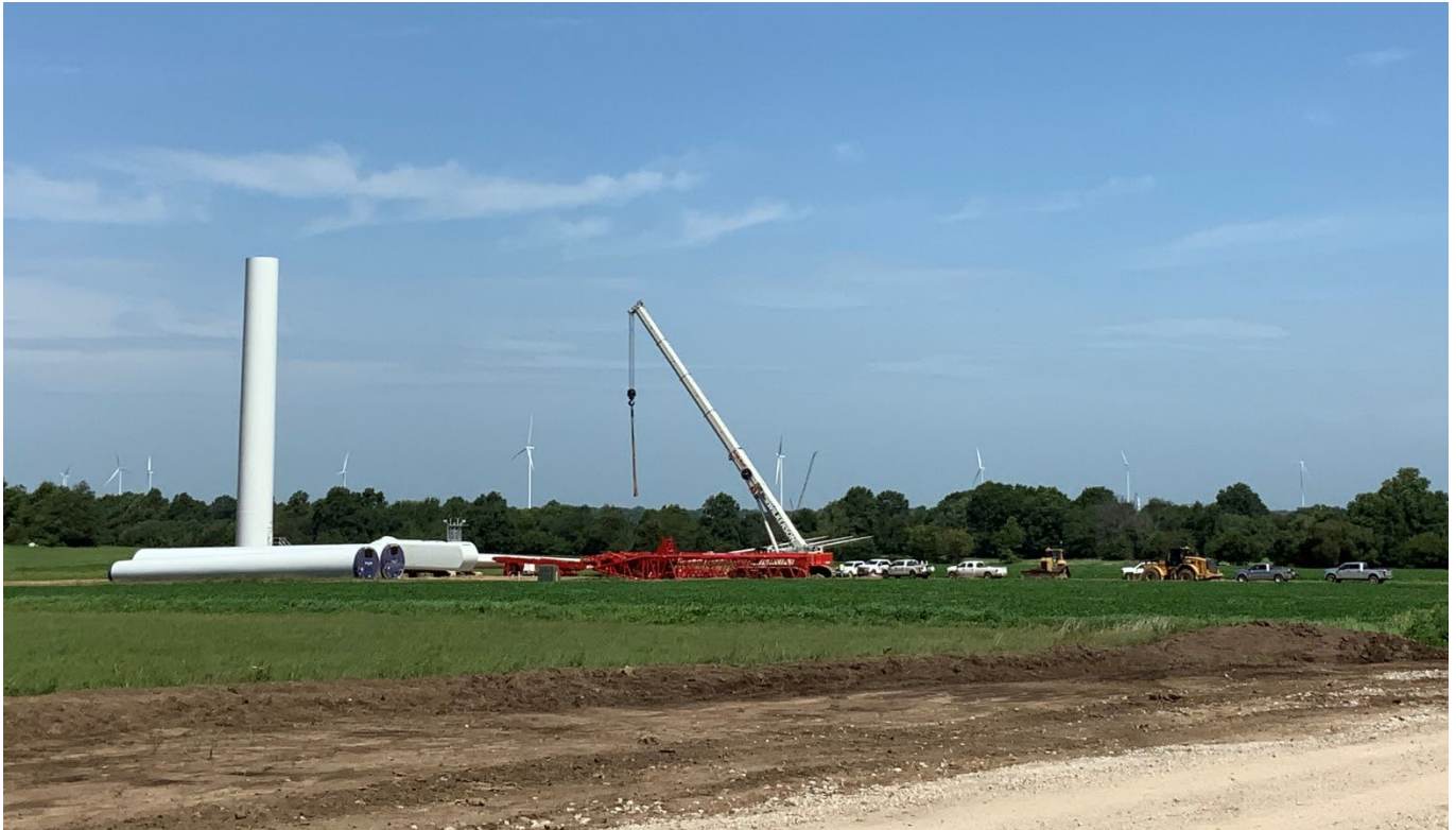
Turbine Pad – Base Section
