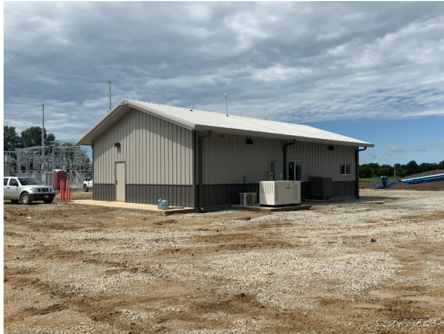
Picture 1. Satellite O&M building (substation in background).
