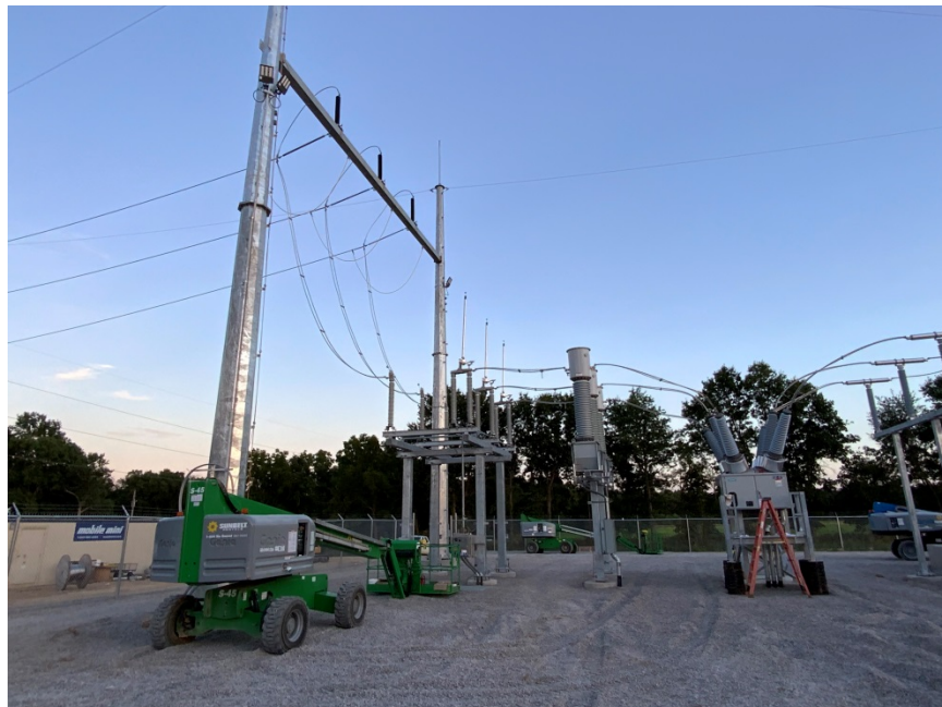
Picture 2. Substation progress photo (July 24 th ).
