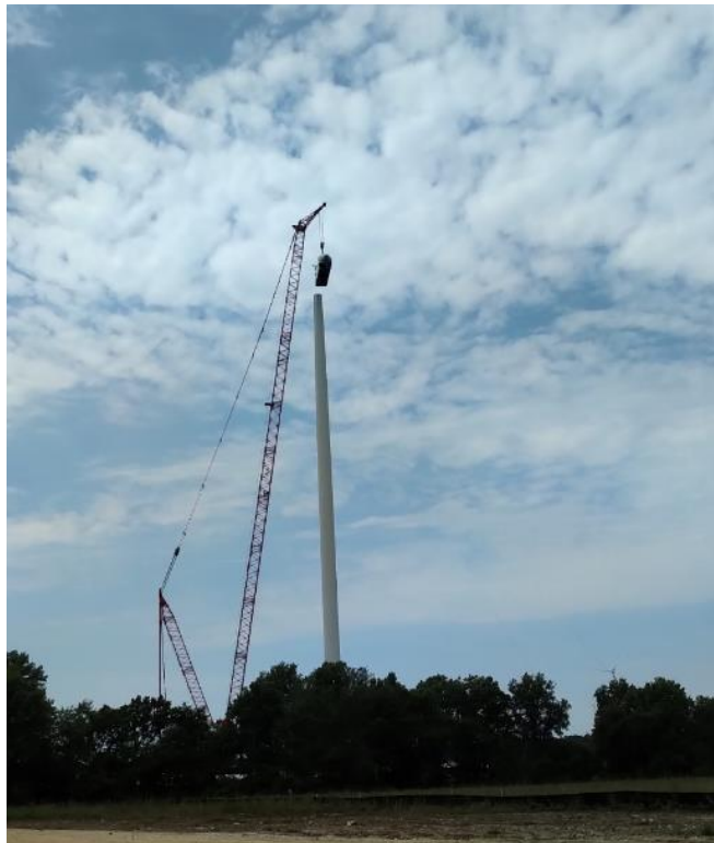
PHOTO 4: NACELLE INSTALL AT T42
