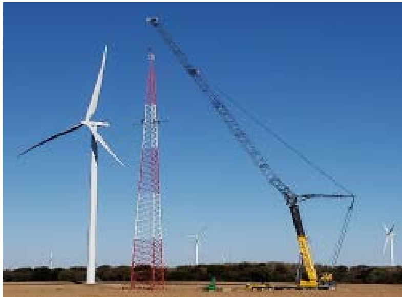
Picture 2. Top out of permanent met tower.
