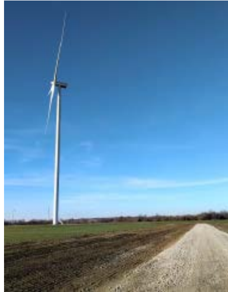
Picture 1. Finished turbine access road and re-vegetation in progress.
