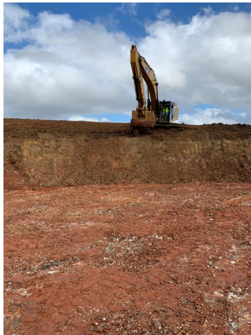
Picture 2. Foundation excavation for T-56.
