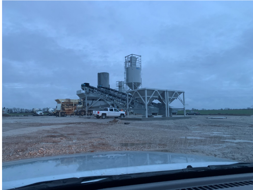
Picture 1. Concrete batch plant.
