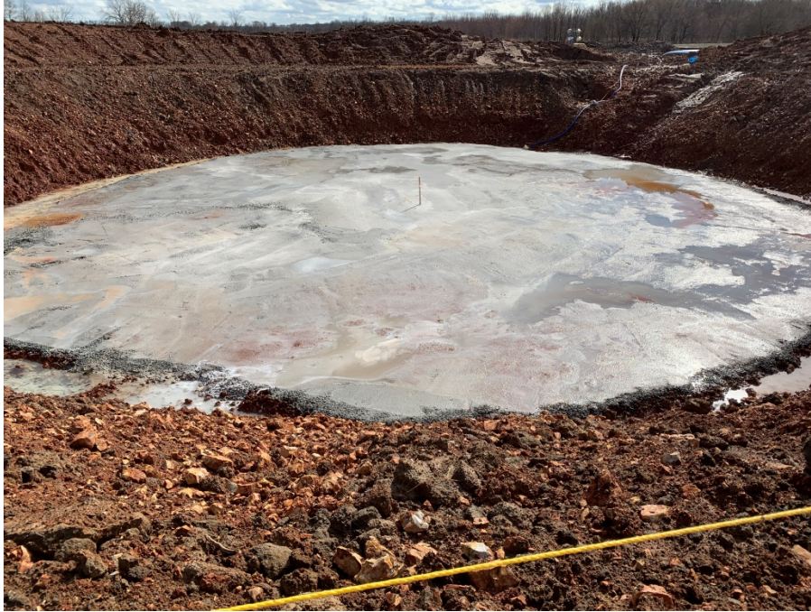
Picture 3. Mud mat in T-62 foundation excavation.
