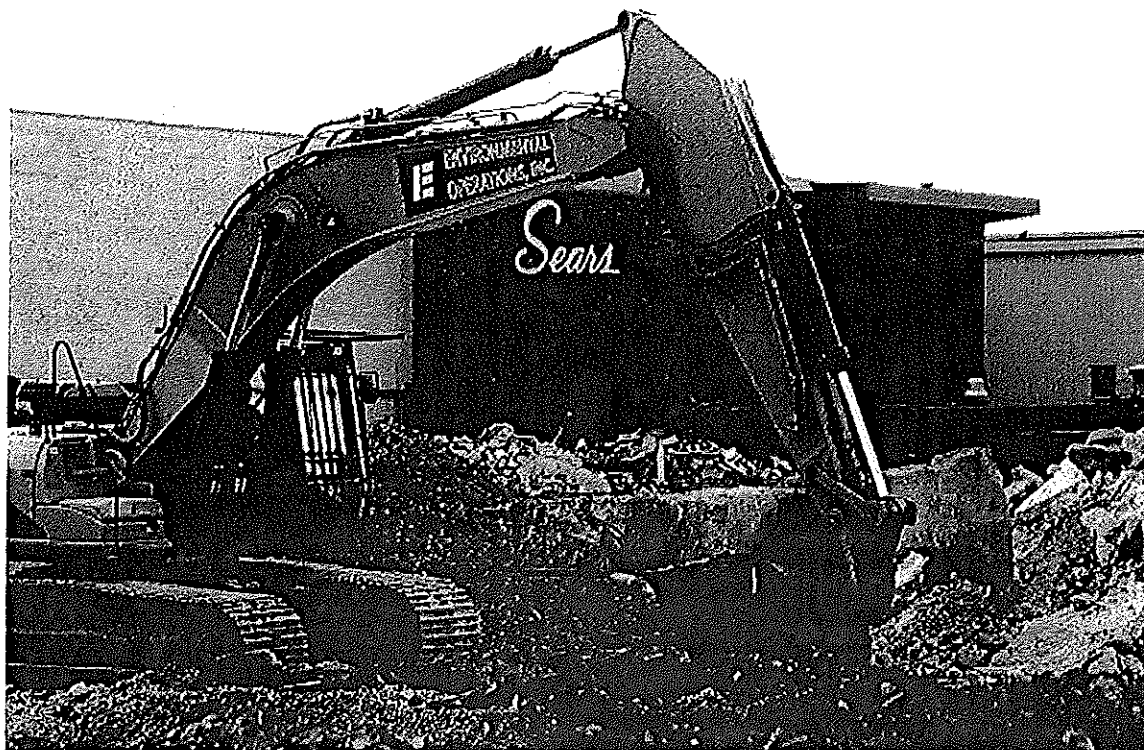
Heavy machinery moves chunks of rubble as demolition continues on portions of Northwest Plaza in St. Ann on Thu 2013. Photo by Christian Gooden, cgooden@post-dispatch.com
